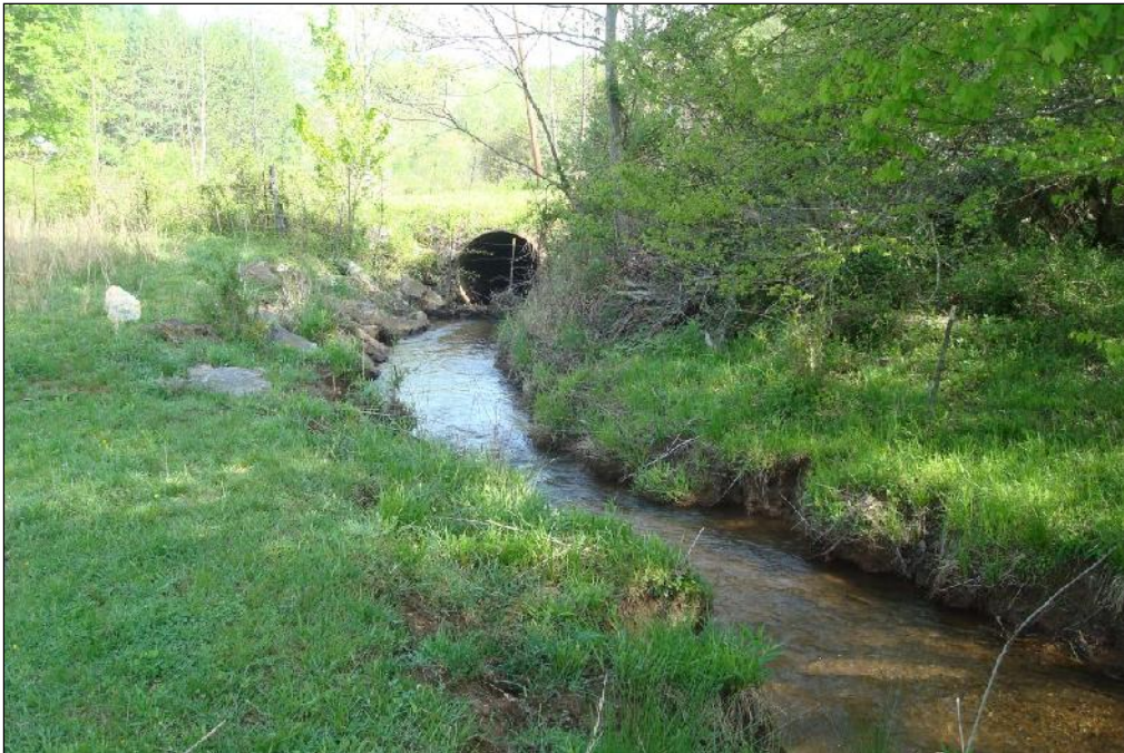
Cochran Branch facing downstream, @ Sta 114+00
