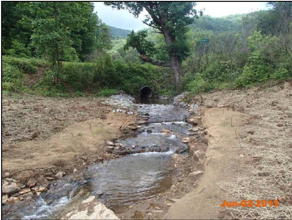
Cochran Branch Reach 1a – Permanent Photo Station 1 Station 101+33 - Upstream
