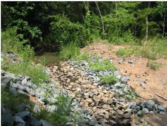
Photo 19 - Upper Reach Sewer Crossing
