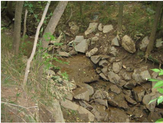
Photo 2 - Lower reach sewer crossing
