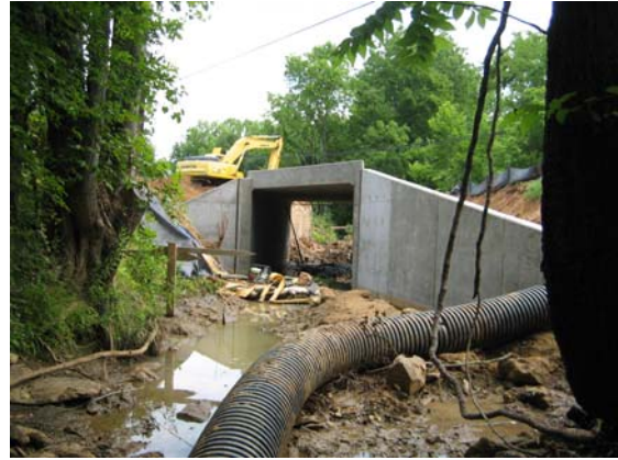
Photo 13 - Culvert Replacement in progress
