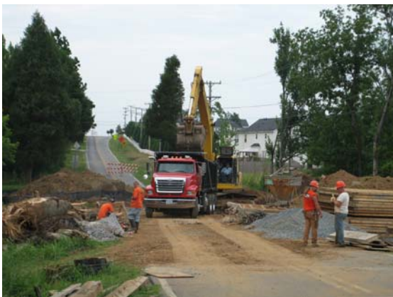
Photo 3 - Culvert replacement on Rocky River Rd.
