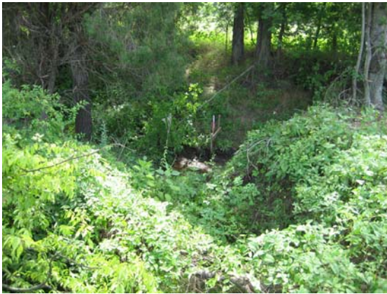
Photo 10 - Trib directly upstream of culvert.
