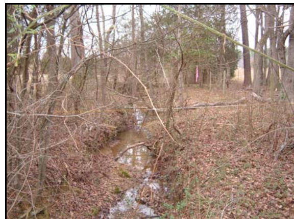
A view downstream of Tributary 1 approximately 100 feet below the culvert.
