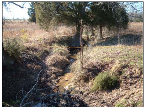
A downstream view of Tributary 1 after the confluence with Tributary 1B.
