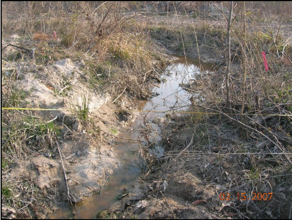
Conoconnara Stream Restoration STA 3+84 Upstream
