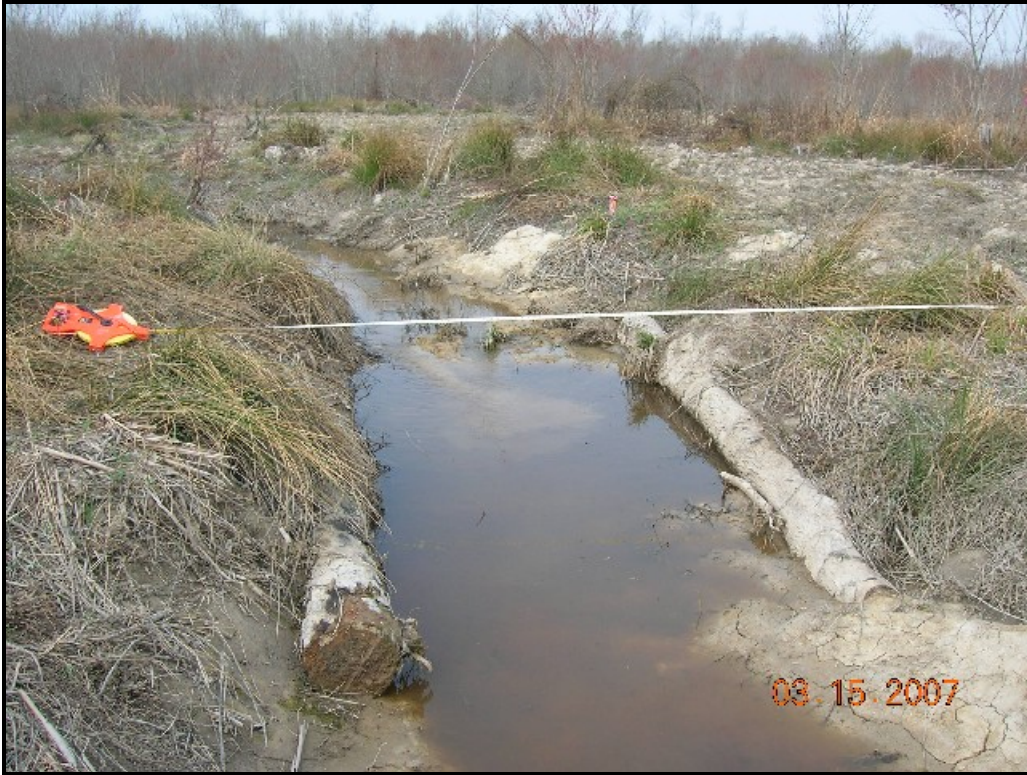
Conoconnara Stream Restoration STA 34+19 Upstream
