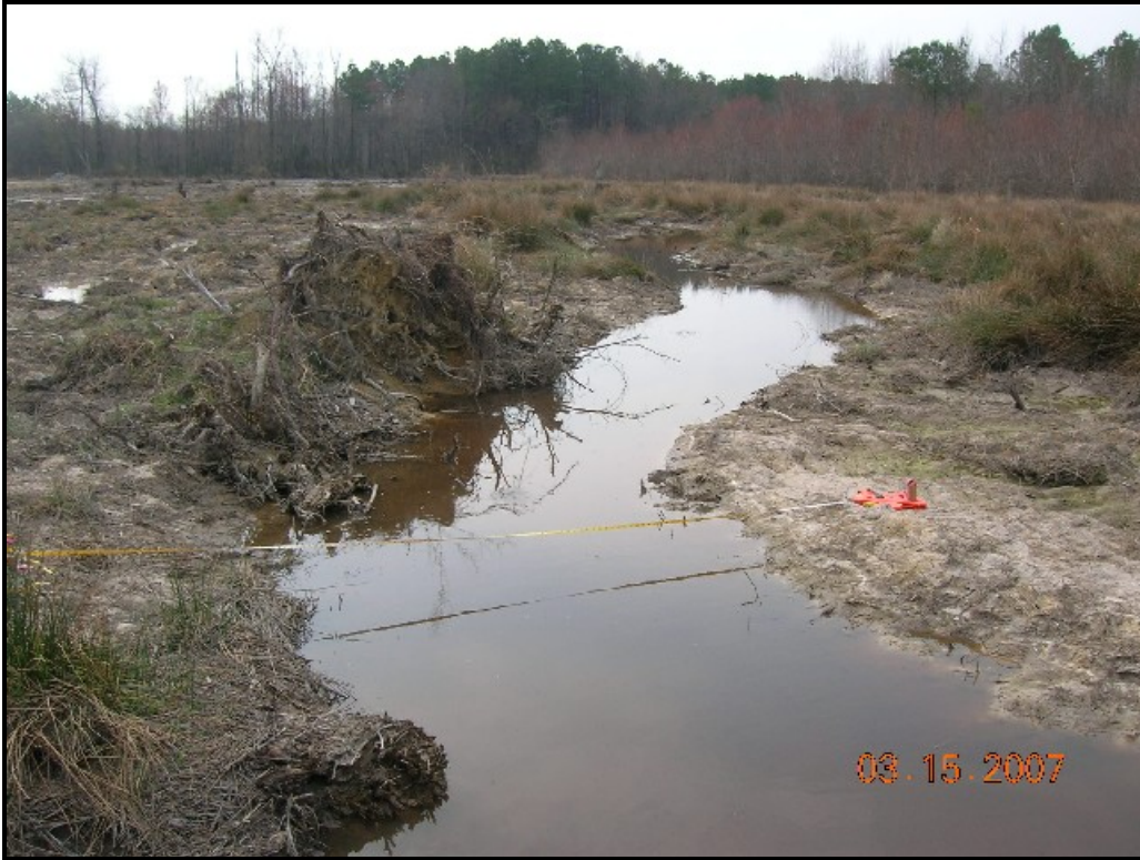
Conoconnara Stream Restoration STA 44+63 Upstream
