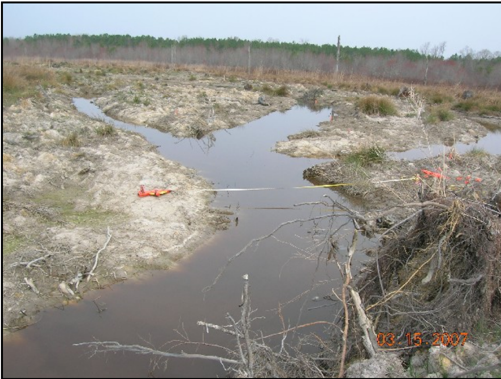
Conoconnara Stream Restoration STA 44+63 Downstream
