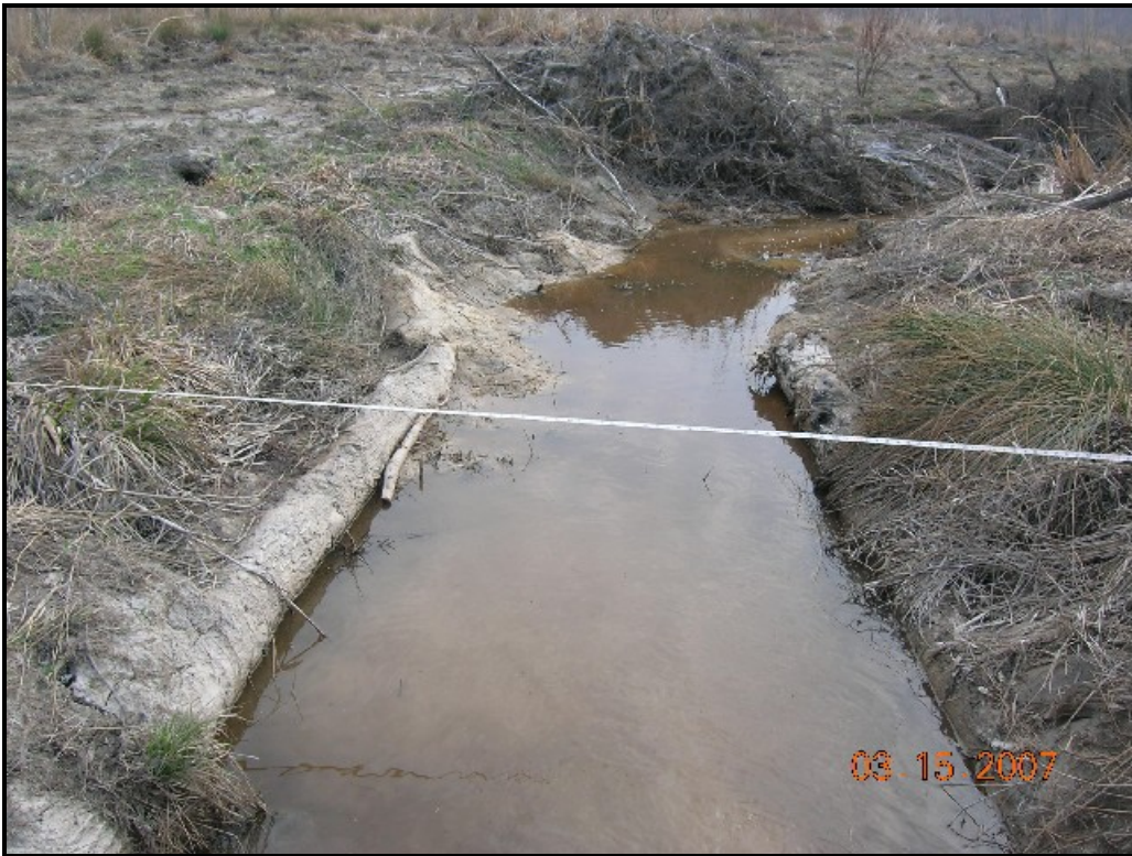
Conoconnara Stream Restoration STA 34+19 Downstream
