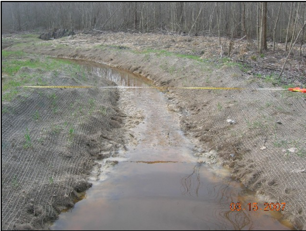
Conoconnara Stream Restoration STA 25+53 Downstream
