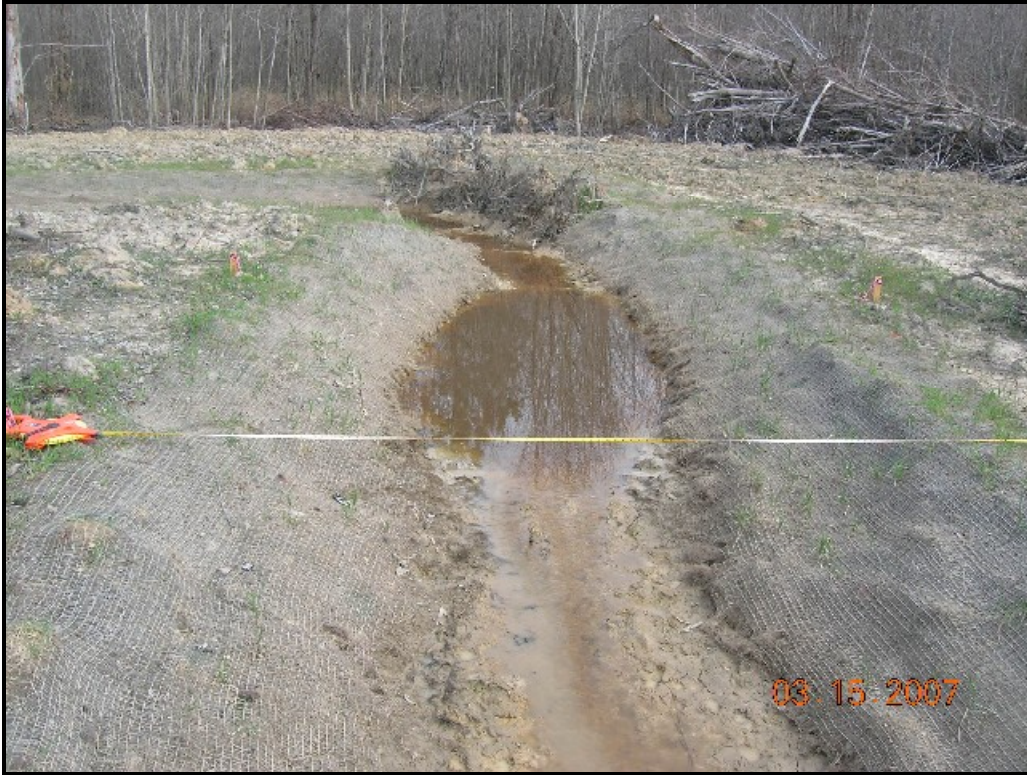
Conoconnara Stream Restoration STA 25+53 Upstream
