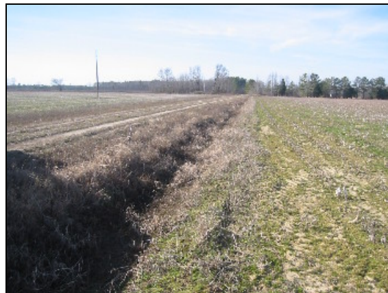
Existing Railroad Bed
