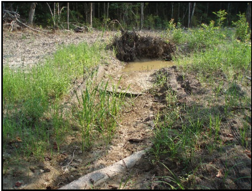
Log grade control and root wad in the bend.
