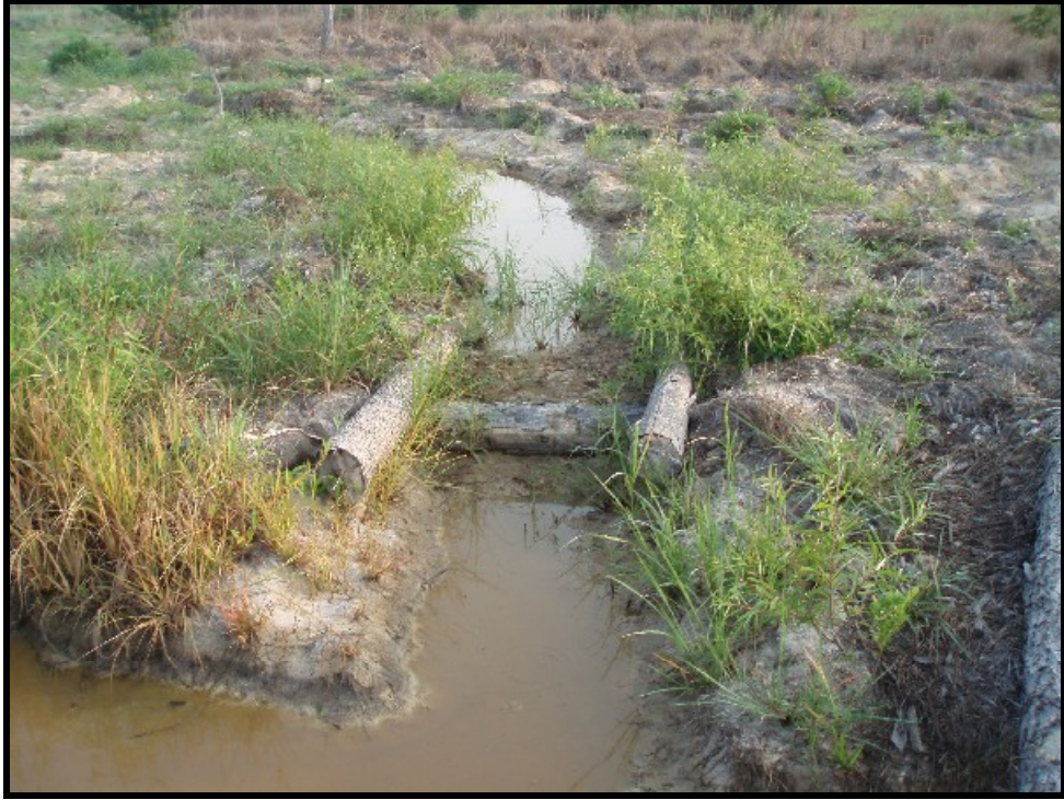
STA 43+25, typical log grade control located at a side channel.
