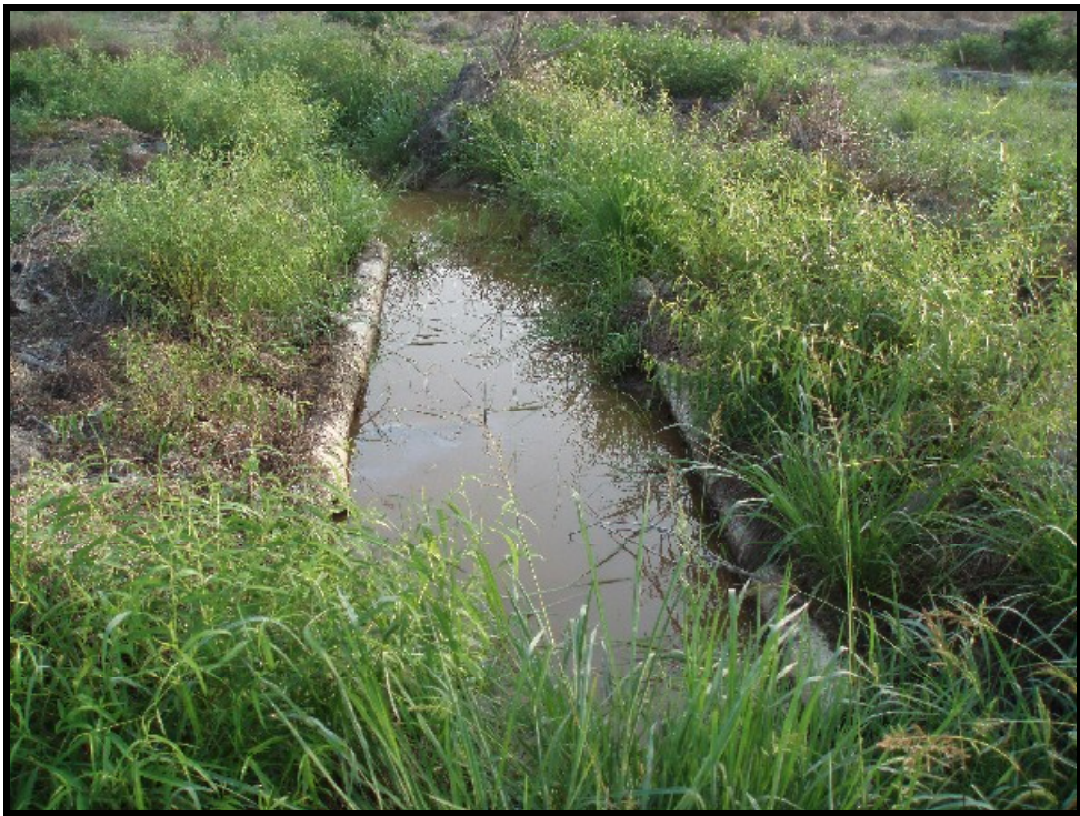
Typical log toe protection structure.
