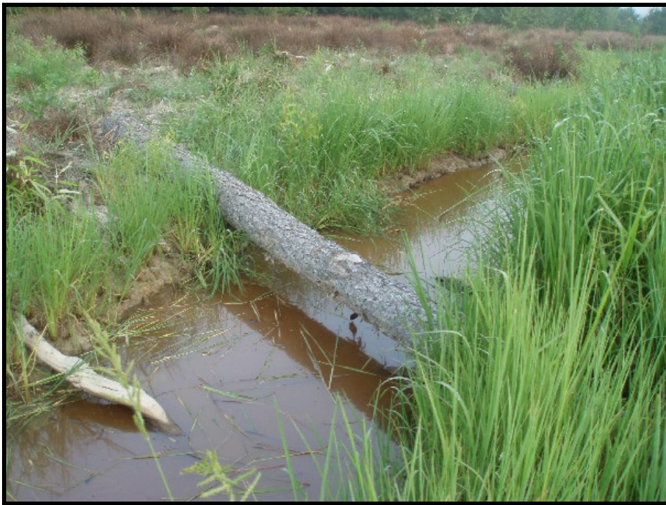
STA 43+30, typical large woody debris found in the channel.
