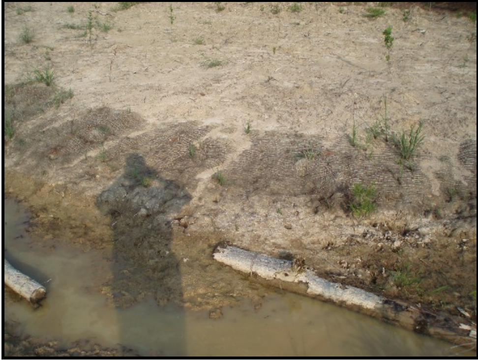
SPA 3. Typical bare bank found along the reach.
