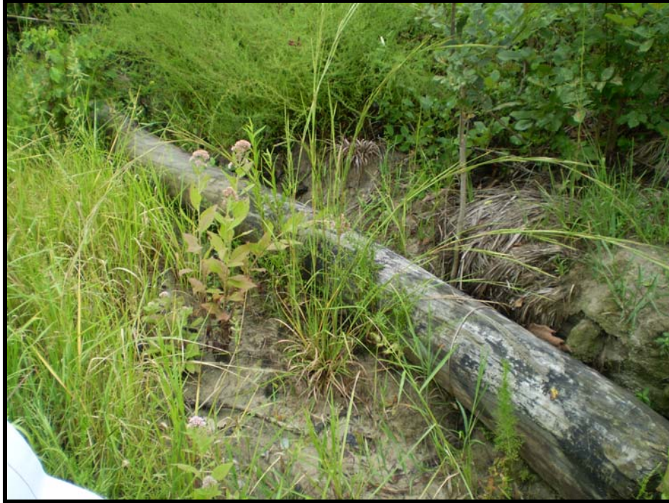
SPA 1. Log toe that washed out away from right bank at station 0+75.
