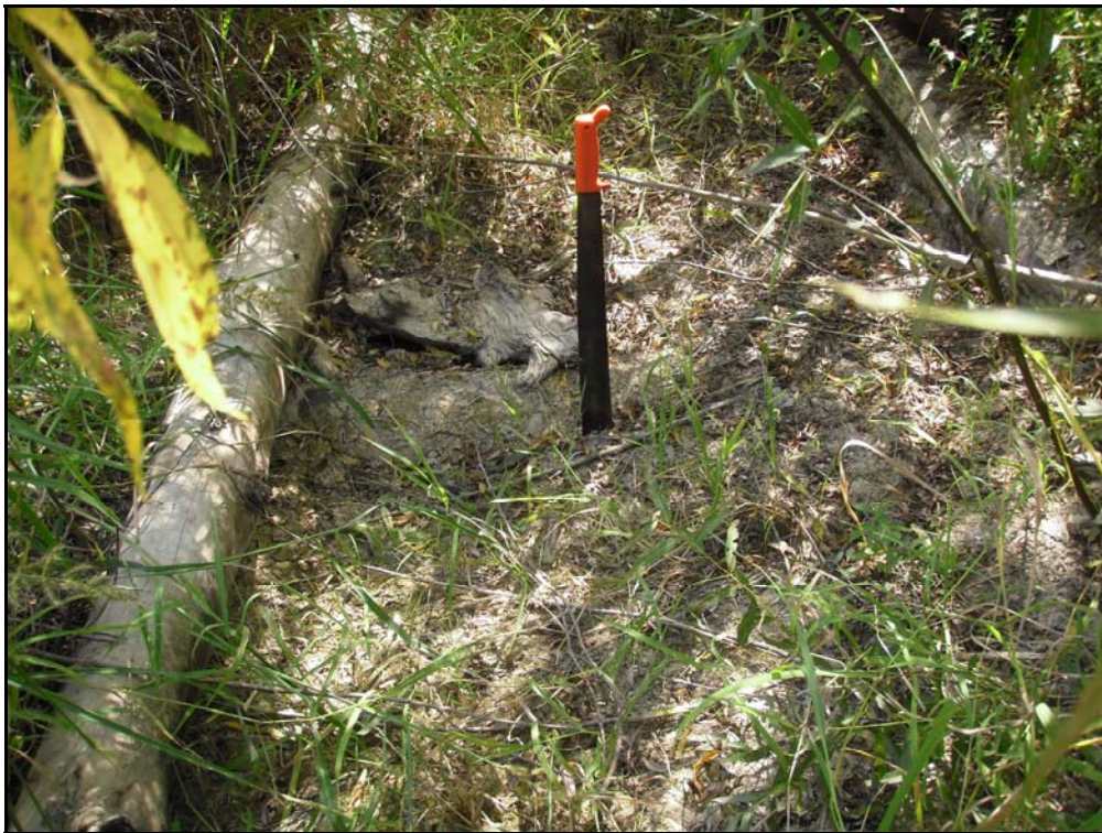
Photo #8 Log Grade Control, Sta. 34+80
