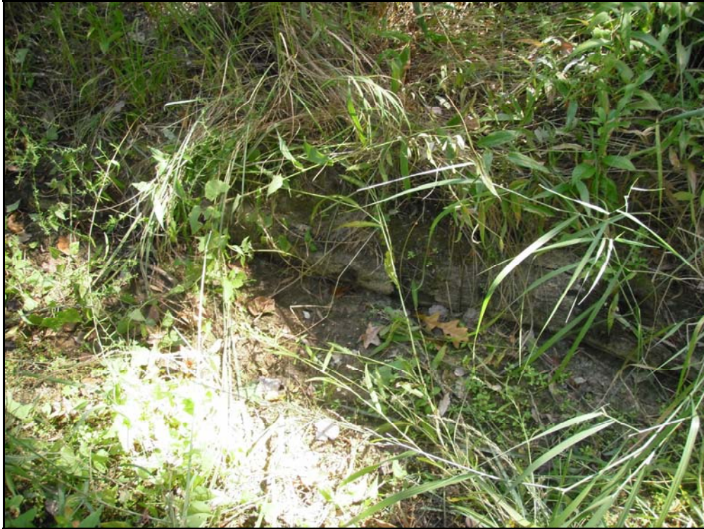
Photo #3 Log Toe, Sta. 11+90
