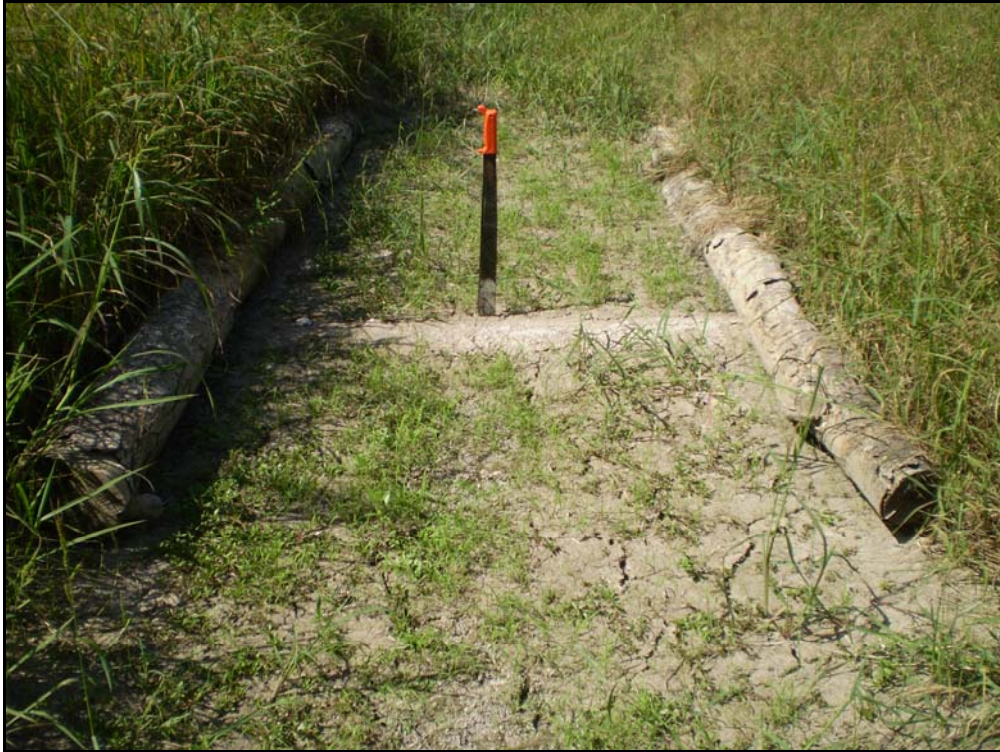
Photo #15 Log Grade Control, Sta. 50+10
