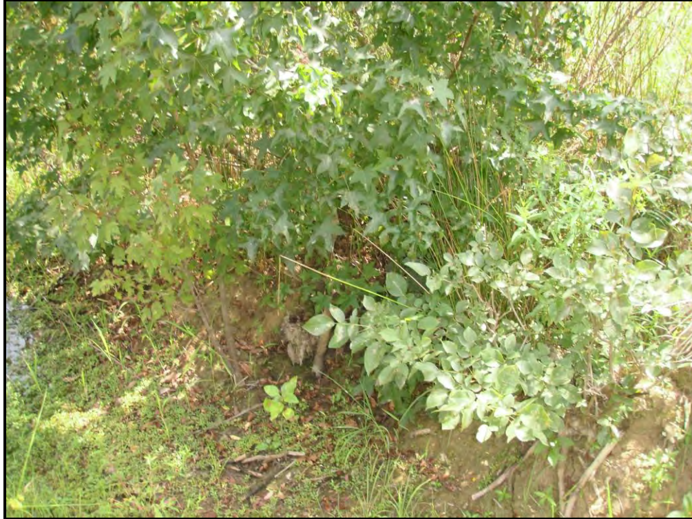
Photo #7 Rootwad, Sta. 31+60
