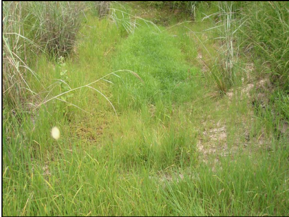
Photo #5 Log Grade Control, Sta. 26+90
