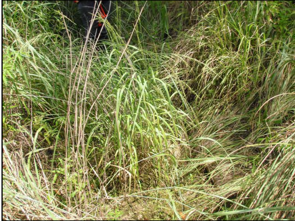
Photo #3 Log Grade Control, Sta. 20+60
