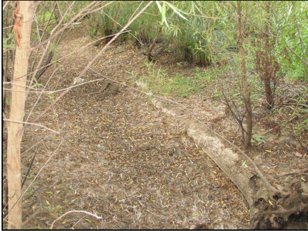
Photo #13 Log Toe, Sta. 43+00
