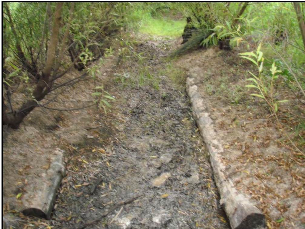
Photo #16 Log Grade Control, Sta.46+25
