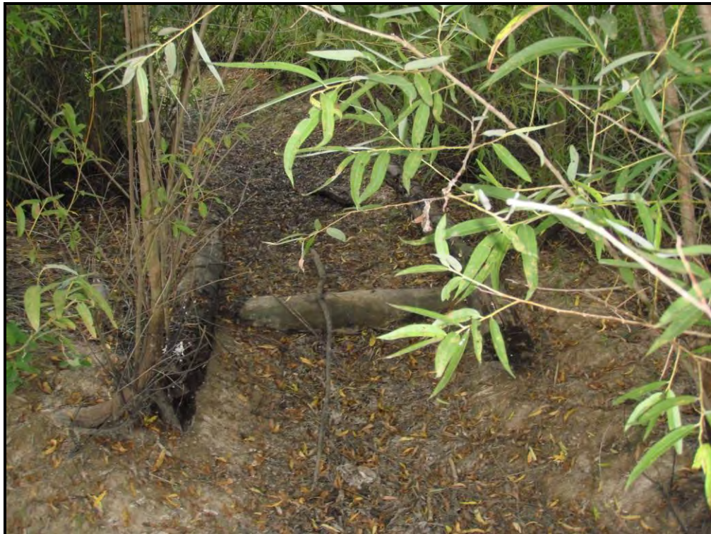
Photo #14 Log Grade Control, Sta. 43+25
