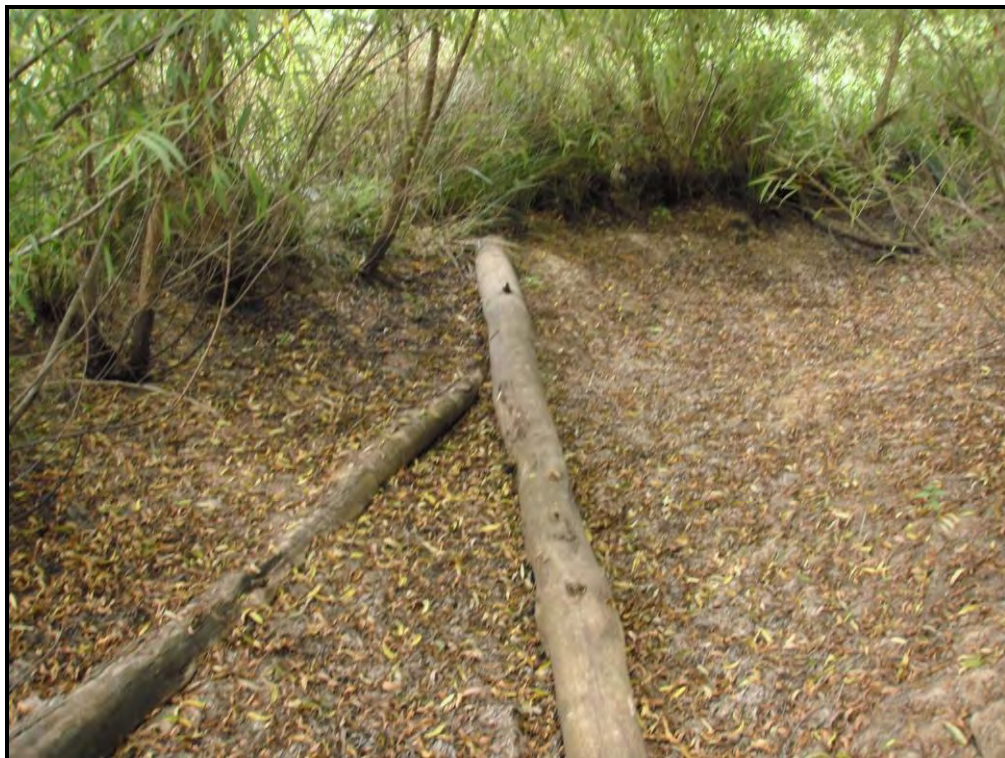
Photo #12 Log Vane, Sta. 39+25
