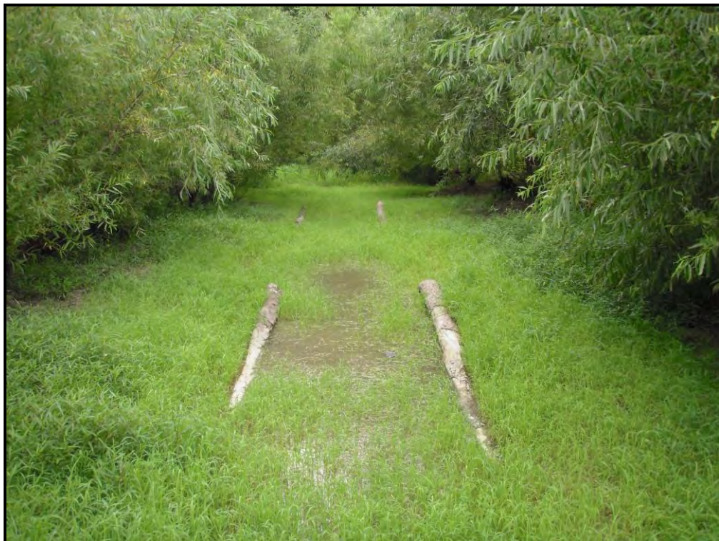
Photo #18 Log Grade Control, Sta.49+00
