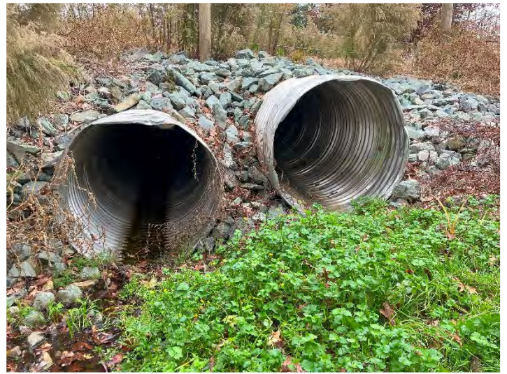
UT to Cedar Creek - Looking Downstream (11/10/2023)
