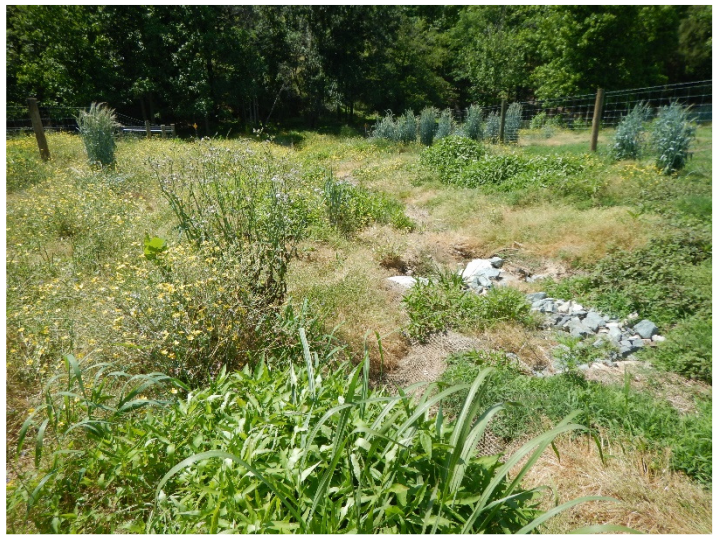
BMP 3 - Facing Downhill (5/12/2023)
