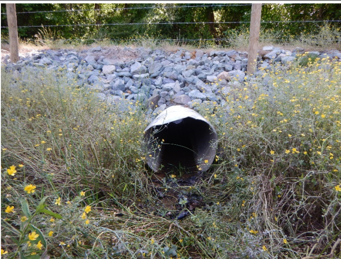
T3 - Looking Upstream (5/12/2023)
