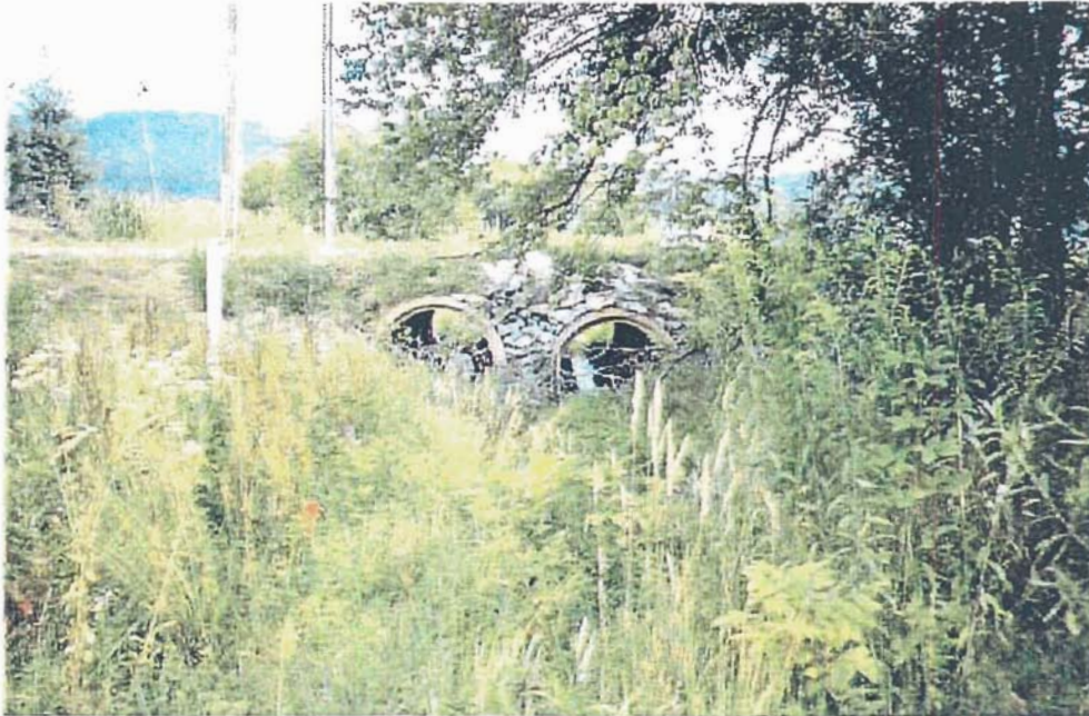
Photo 7: 2-60" RCP at end project (Fairway Falls Rd.)
