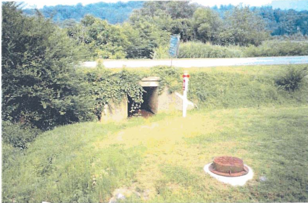
Photo 3: Box Culvert at NC 191
