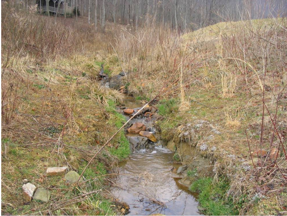
STA 10+80 Looking Upstream at Steep Riffle and Bank Erosion on Left Bank
