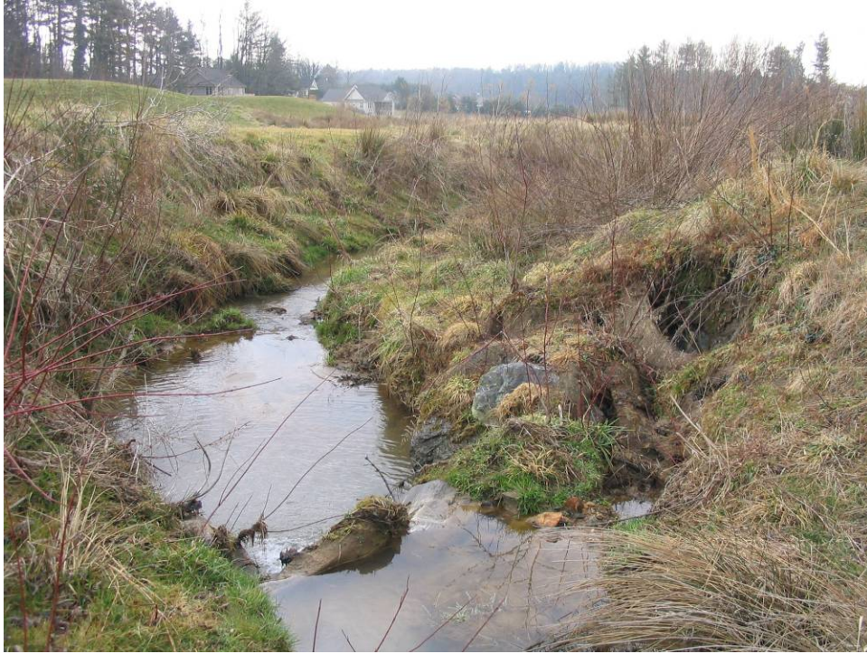
STA 24+25 Looking Downstream at Rock Vane with Right Bank Erosion
