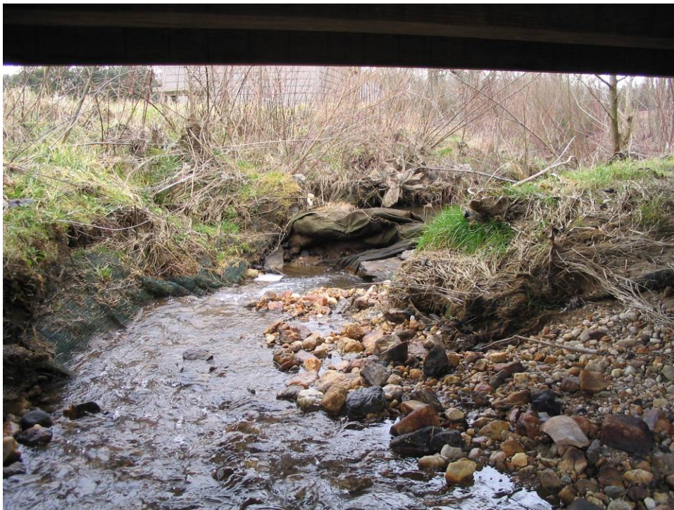
STA 34+90 Looking Downstream at Failed Rock Cross Vane
