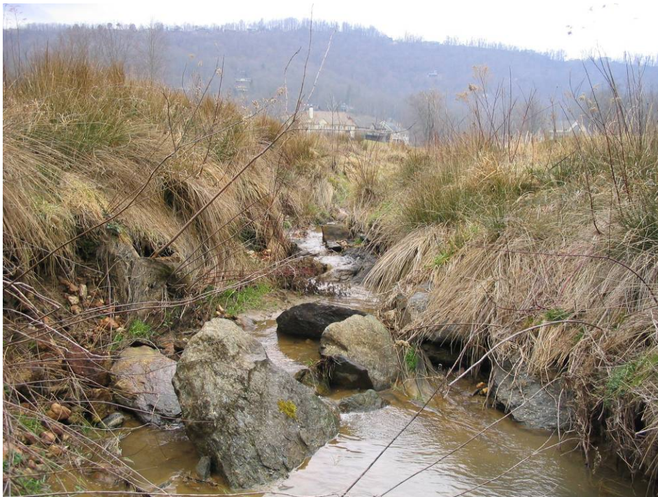
STA 28+20 Looking Upstream at Water Piping Through Rock Cross Vane
