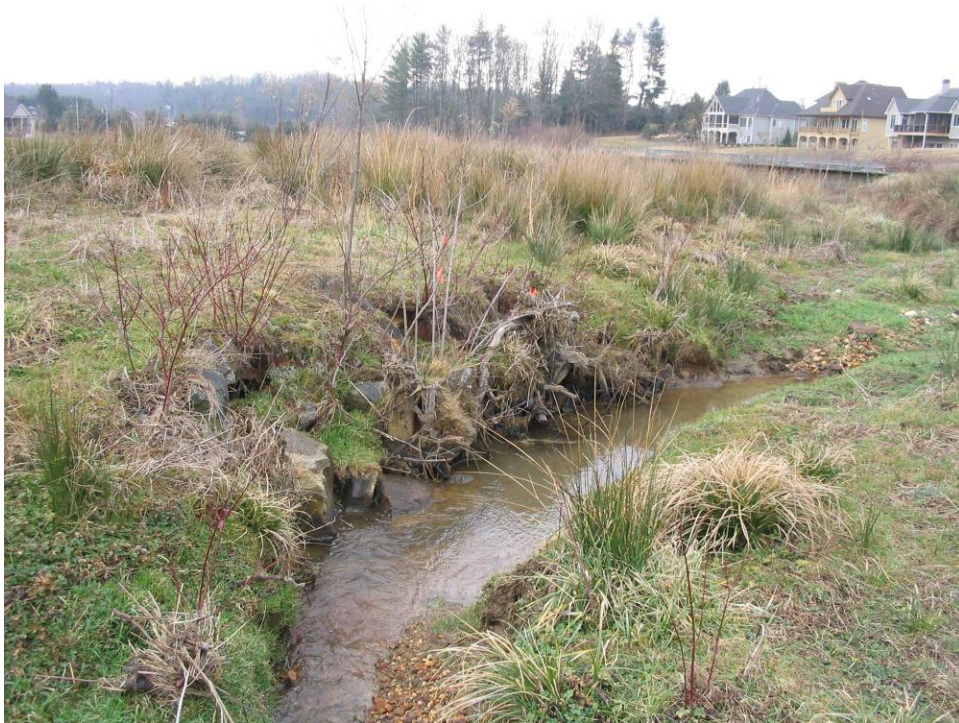
STA 27+30 Looking Downstream at Pool Root Wad with Bank Erosion
