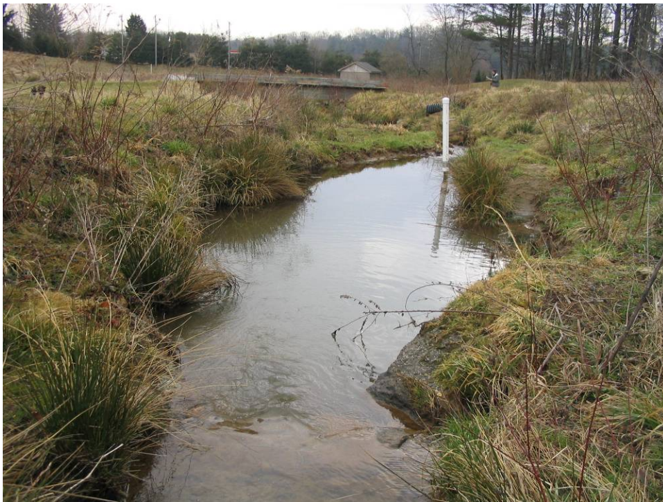
STA 32+20 Looking Downstream at Scour Pool and Rock Cross Vane
