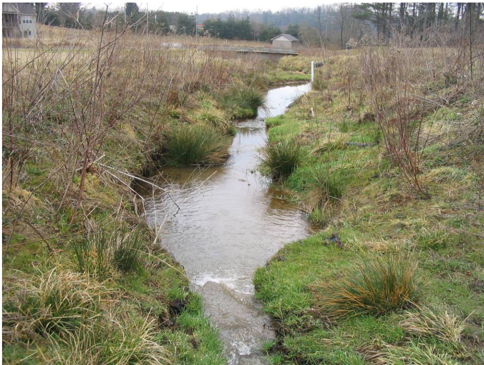
STA 31+80 Looking Downstream at Scour Pool and Rock Cross Vane
