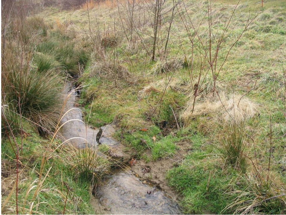
STA 13+20 Looking Downstream at Water Piping Through Rock Cross Vane
