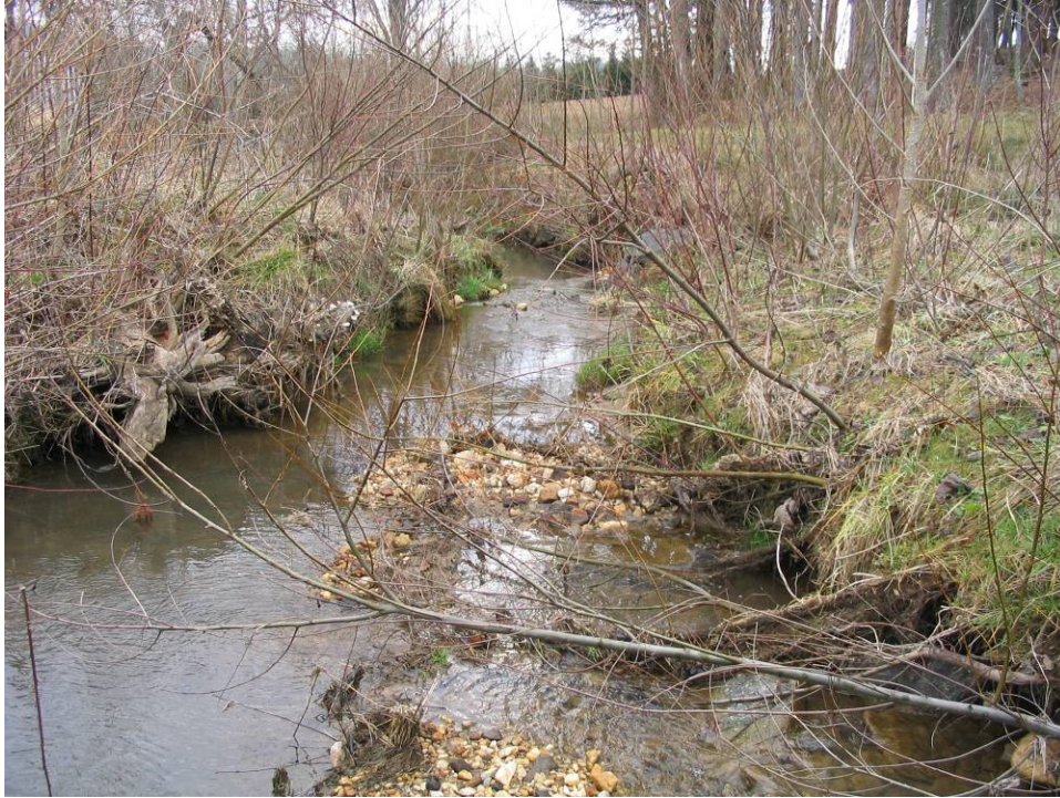
STA 35+10 Looking Downstream Bank Erosion and Slumping
