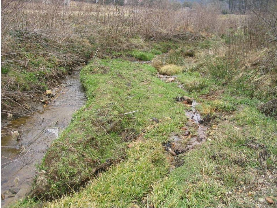
STA 31+70 Looking Downstream with Chute Cut-Off Forming
