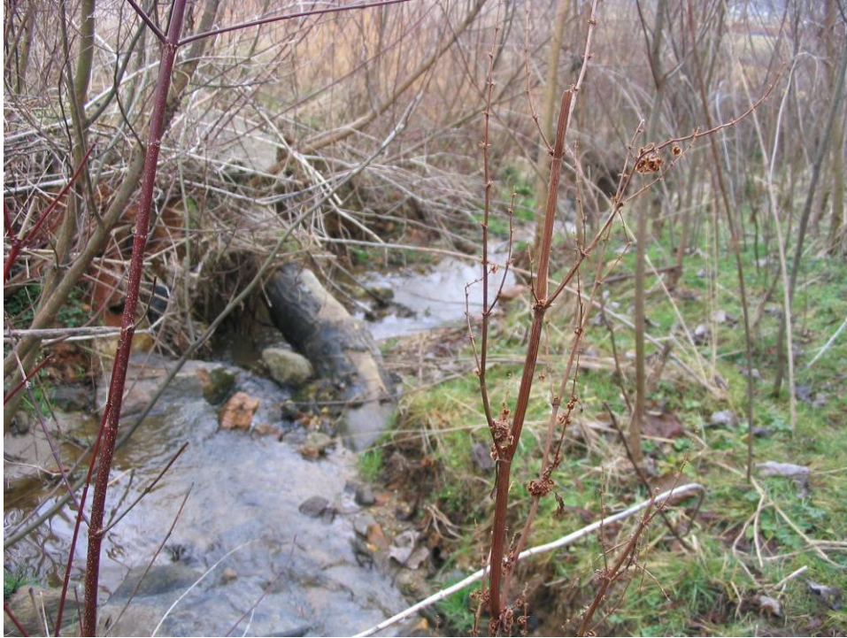
STA 20+45 Looking Downstream at Undercut Log vane
