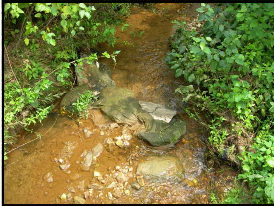
Figure 3—Typical Failing Structure
