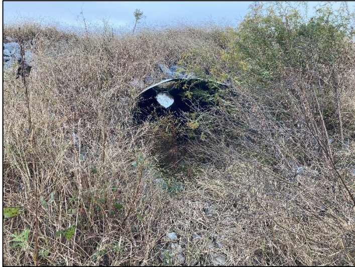
Photo Point 1: Culvert at the bottom of KJ1-B (11/3/2022)
