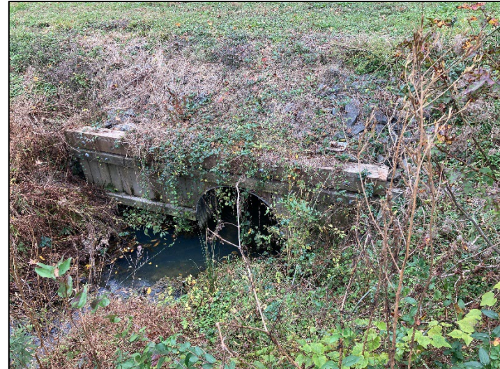
Photo Point 4: Culvert at Kinston Highway (11/3/2022)
