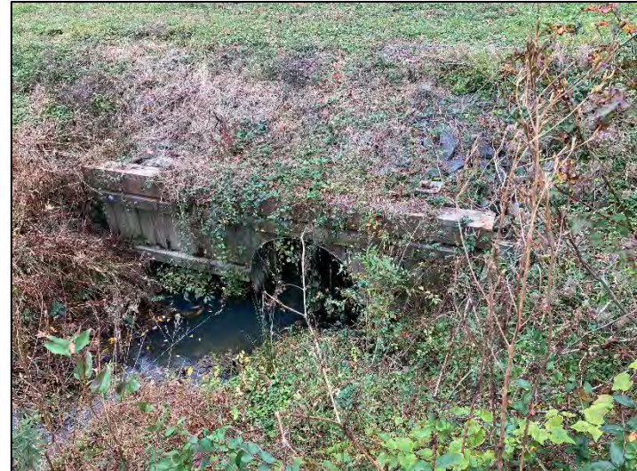
Photo Point 4: Culvert at Kinston Highway (11/3/2022)
