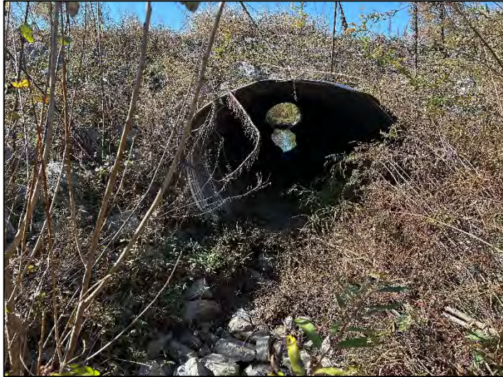
Photo Point 1: Culvert at the bottom of KJ1-B (11/2/2023)
