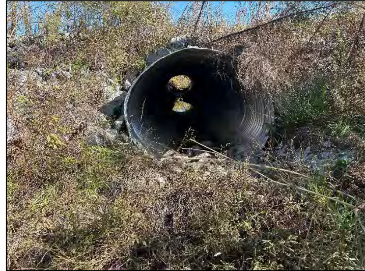
Photo Point 2: Culvert at the top of KJ1-C (11/2/2023)
