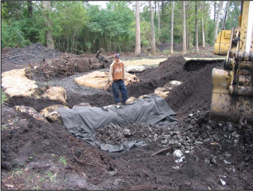
Downstream Invert on a Constructed Riffle
