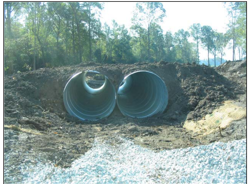
Culvert Installation in Progress
