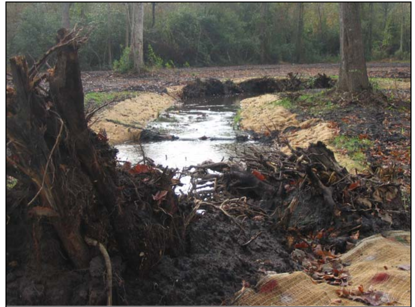
Rootwads & Constructed Riffle
