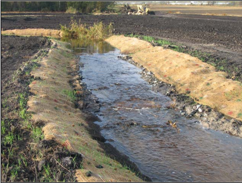
Constructed Riffle
