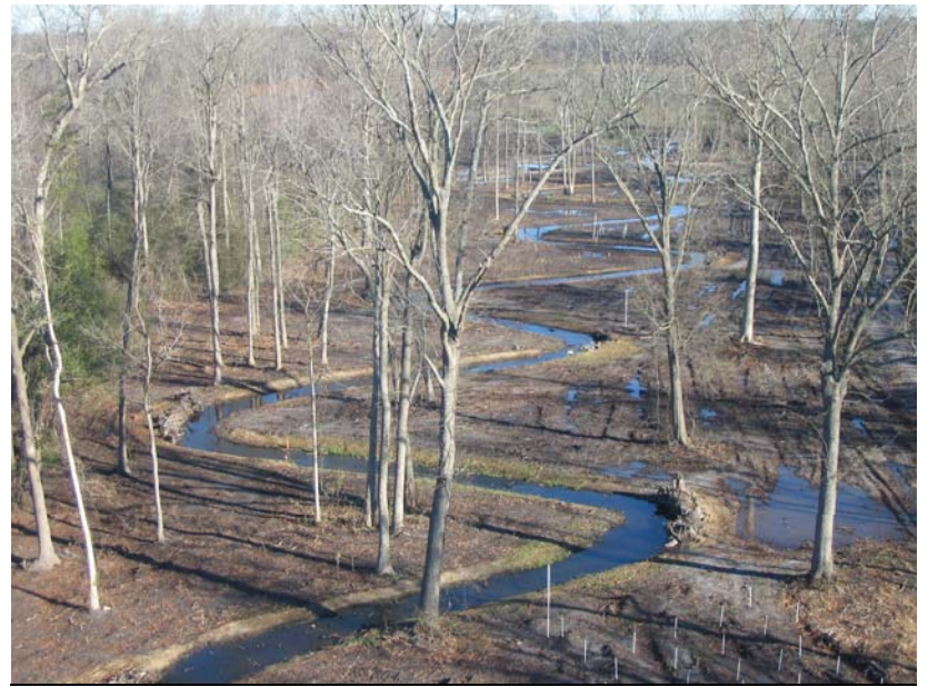
New Stream Channel Routed Through Trees
