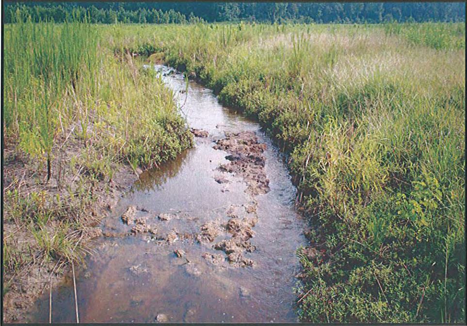
SPA 5. Erosion and bar formation at STA 74+80.
