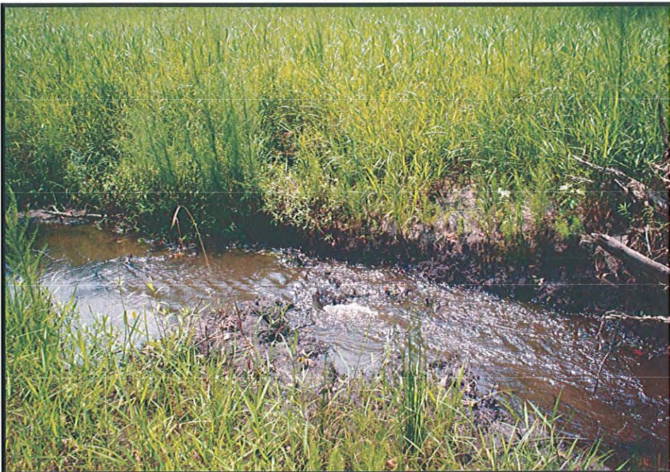
SPA 3. Left bank erosion at STA 51+70.
