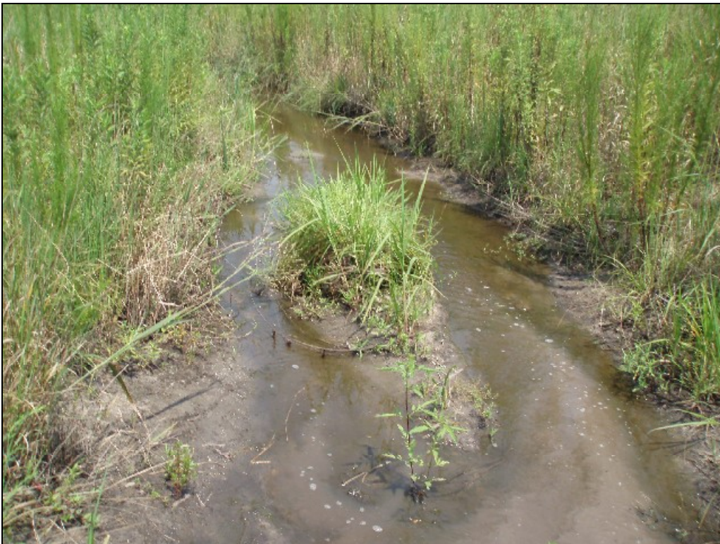
SPA #12. STA 59+20. Bed erosion and mid-channel bar formation.
