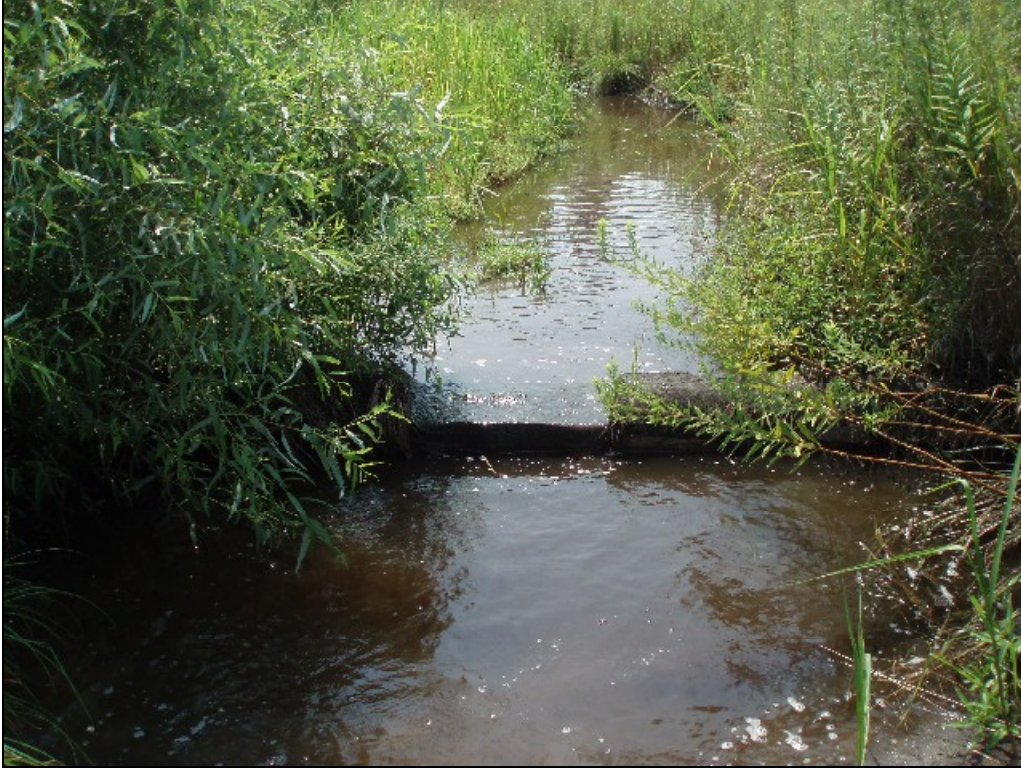
SPA #11. STA 59+10. Log weir end cut on right bank.
