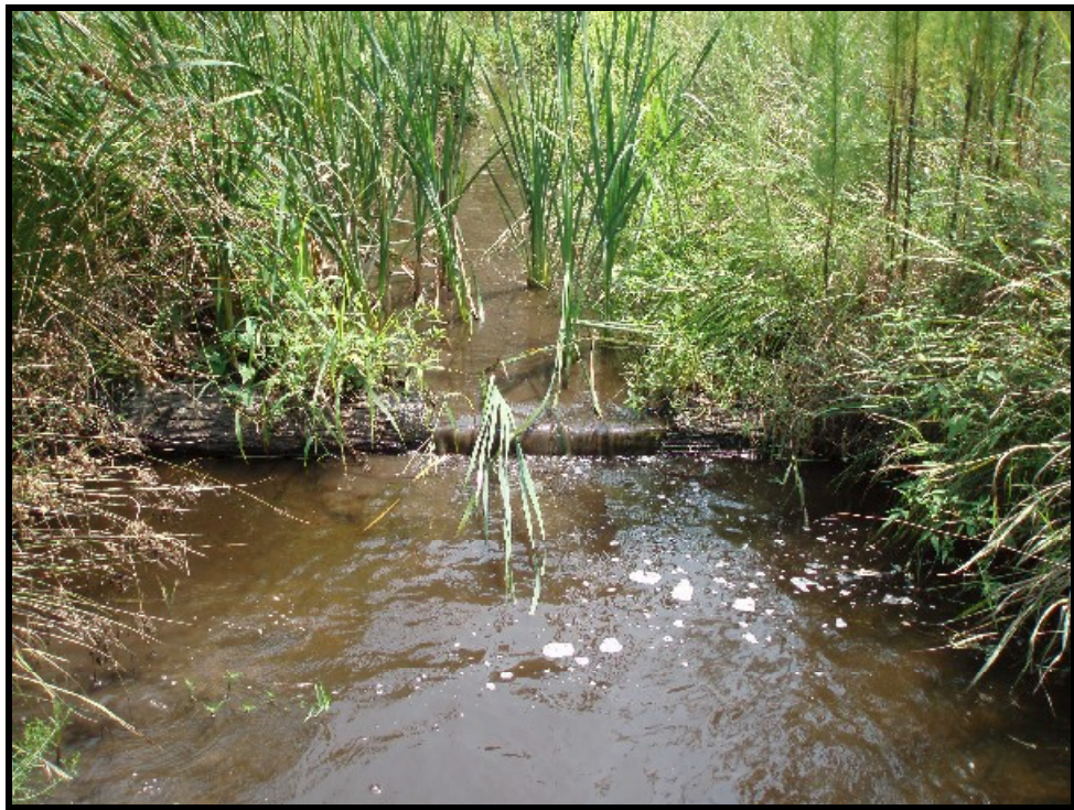
Photo 2. Typical log weir, installed correctly.
