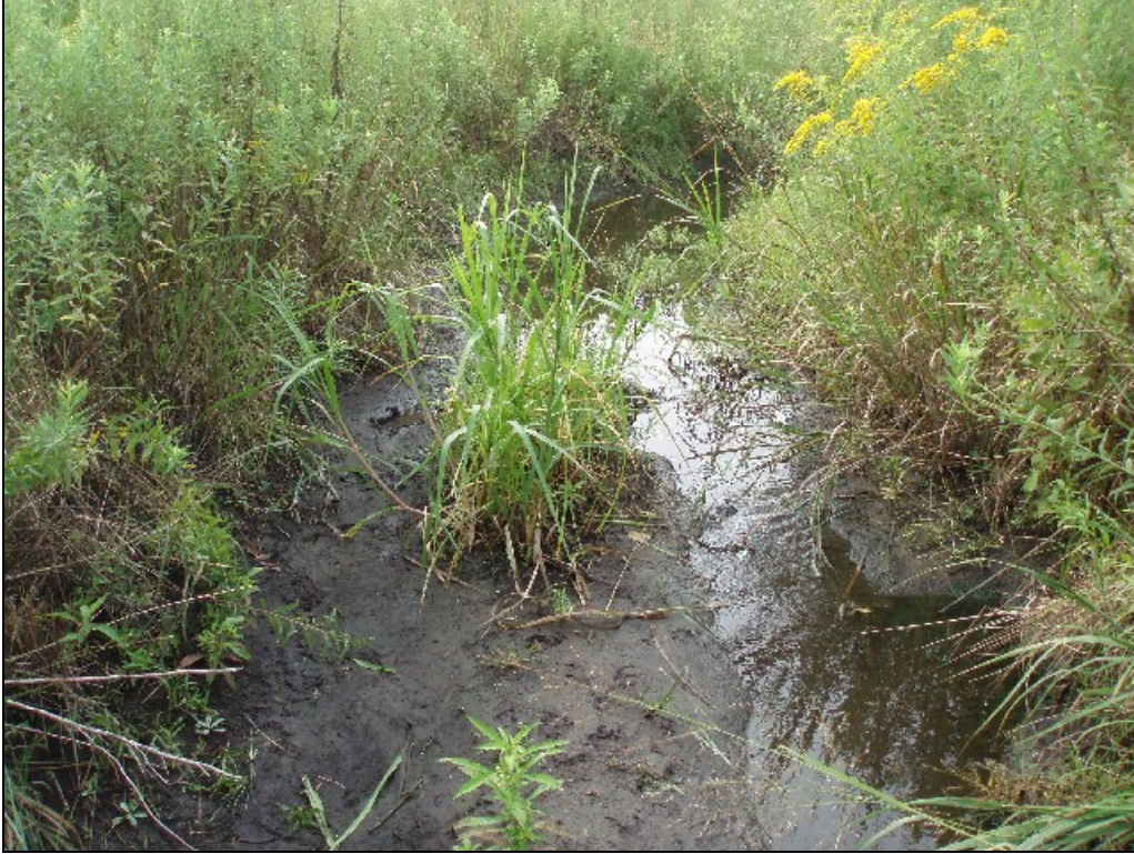
SPA #13. STA 63+00. Bed erosion and mid-channel bar formation.
