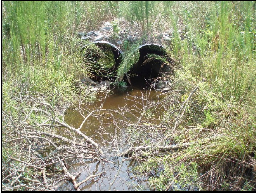
Photo 3. Typical double barrel corrugated metal pipe culverts and stream crossing.
