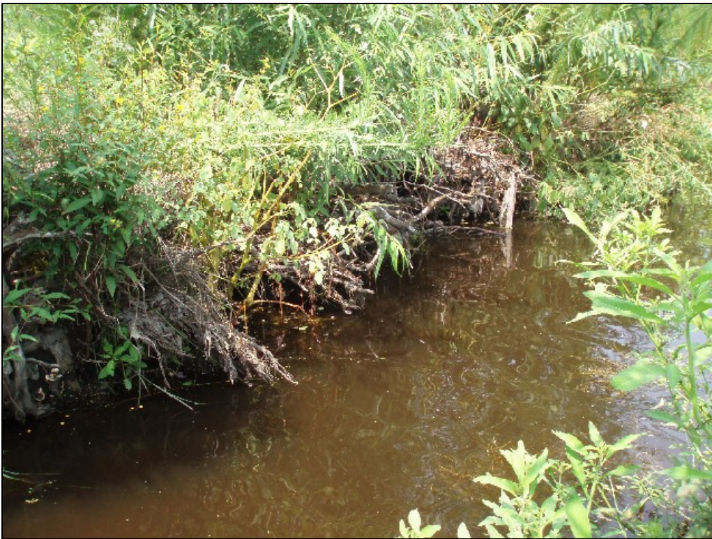
SPA #2. STA 23+50. Erosion on left bank behind rootwad.
