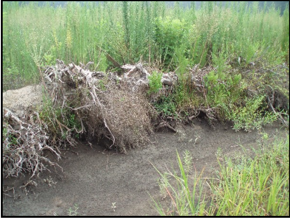
Photo 9. Typical root wad structures to armor bends.
