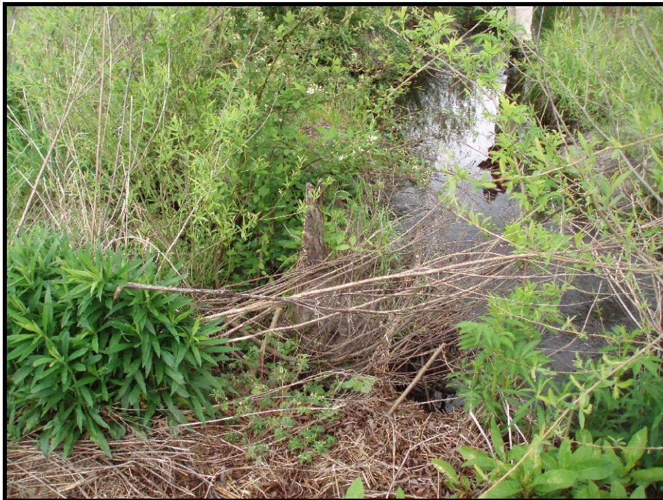
SPA6. Sta. 25+40 Erosion on left bank behind root wads.
