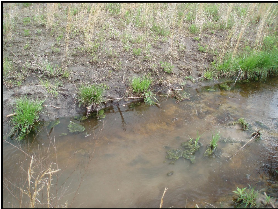
SPA12. Sta.74+50 Erosion downstream of log vane due to improper installation; planted with live stakes to stabilize banks.
