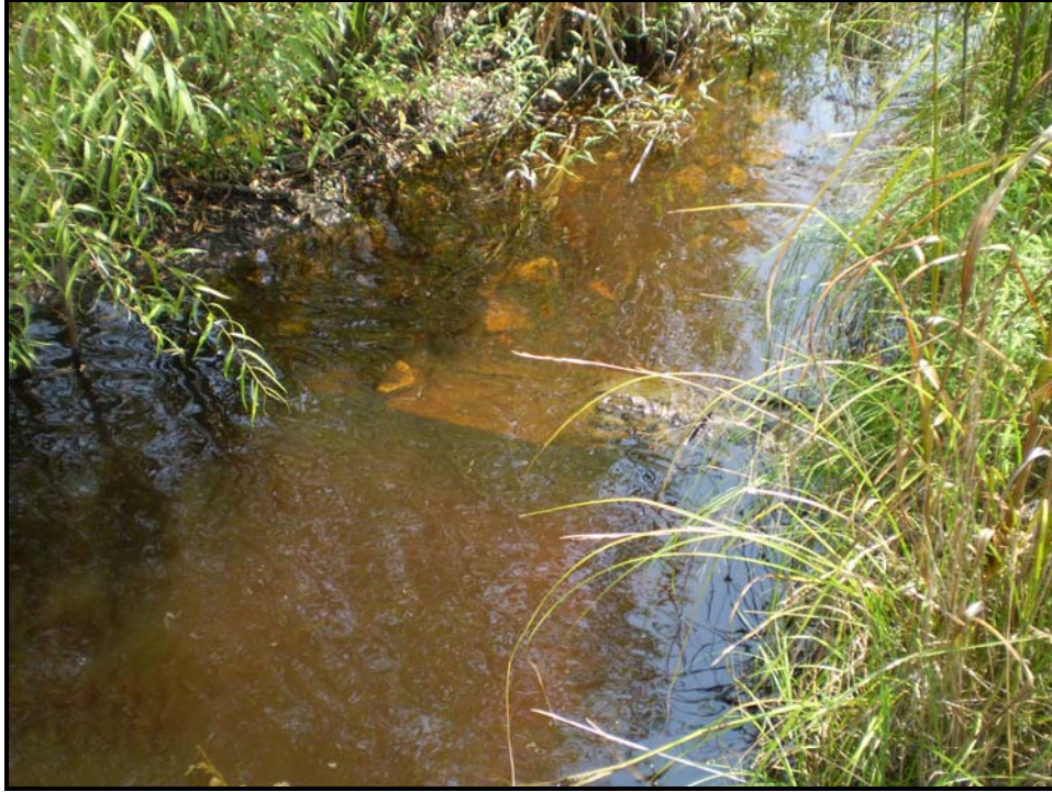
SPA 7 – Erosion at log weir, Sta. 76+90.
