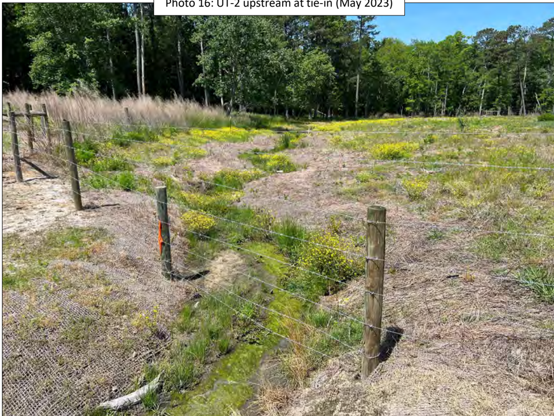
Photo 16: UT-2 upstream at tie-in (May 2023)
