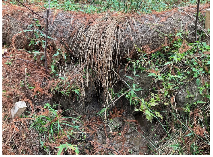
Repaired Wetland Headcut (11/10/2022)
