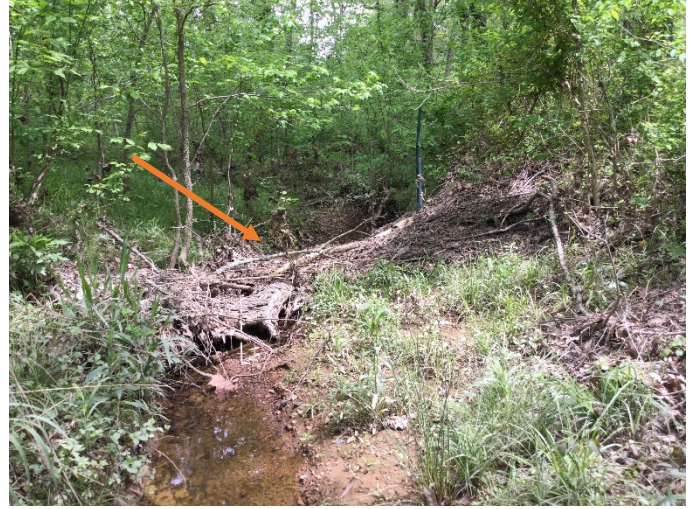
Wrack Lines – UT2 (4/18/2022)
