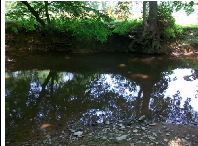
Photo 15-View of Crooked Creek XS2 Pool, facing left bank.
