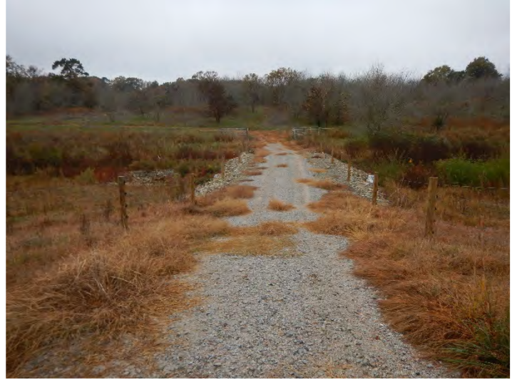
UT1B Culvert Crossing - Looking East (10/26/2022)
