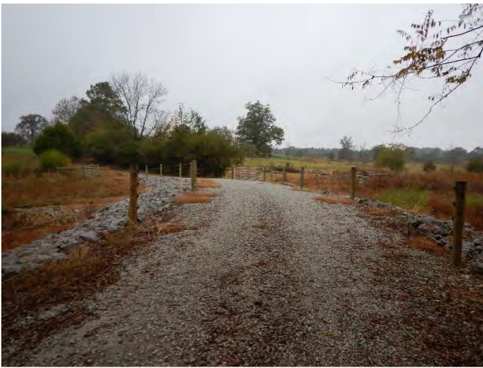
UT1 R2 Culvert Crossing – Looking Southwest (10/26/2022)
