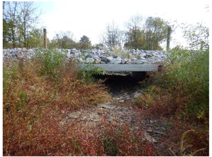
UT1 R2 - Looking Downstream (10/17/2022)
