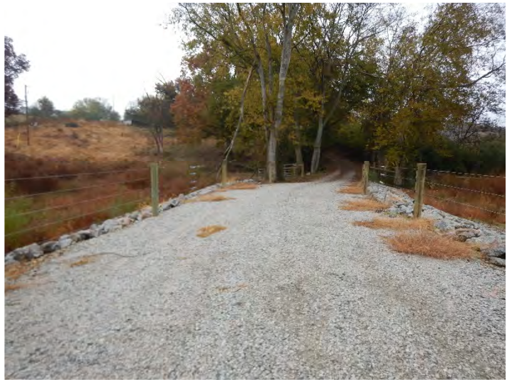
UT1 R2 Culvert Crossing – Looking Northeast (10/26/2022)
