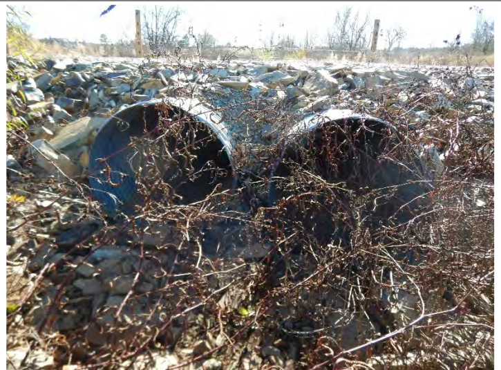
UT1B - Looking Downstream (11/21/2022)
