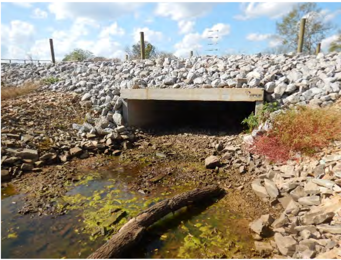
UT1 R2 - Looking Upstream (10/17/2022)
