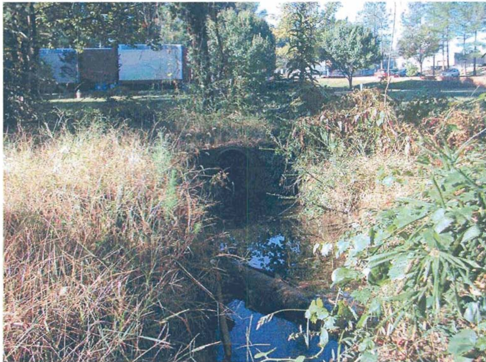
Picture 14. Small drainpipe from Blue Street on south side of property.
