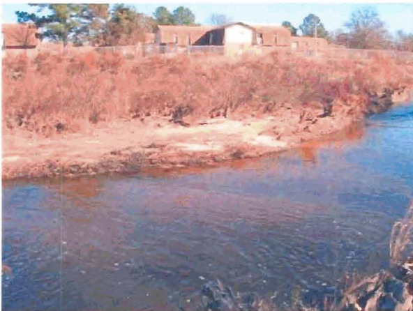
VPA3. Vegetation failure near Station 21+60
