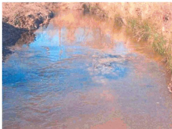
SPA 9. Station 14+20 on LCC. Transverse bar formation and concomitant erosion on left bank.
