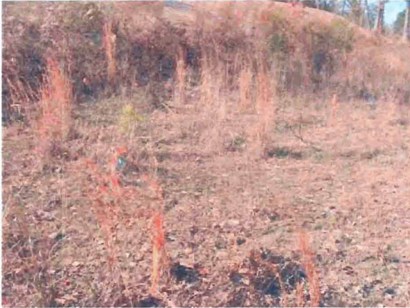
VPA1. Vegetation failure near Station 18+70
