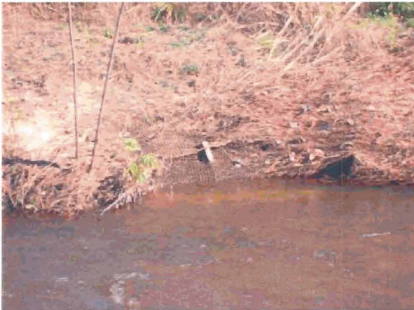
SPA 3. Station 18+50 Bowling effect caused by pool formation below sill.
