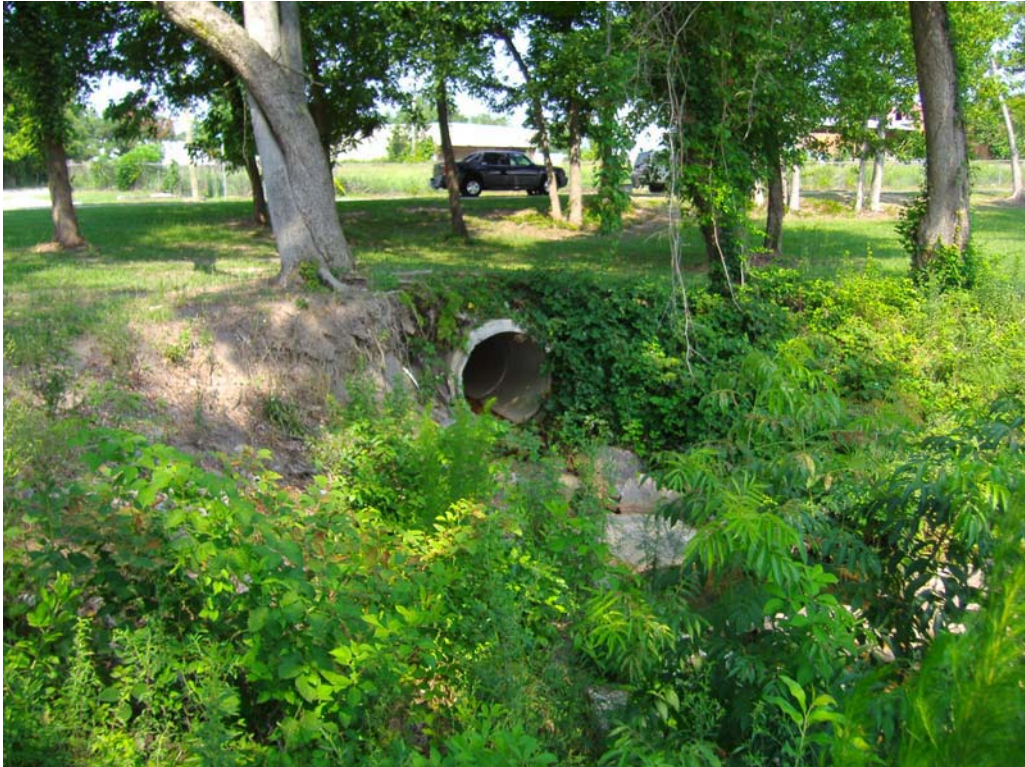
Photo 1. (SP 9) Stormwater outlet pipe entering into the design plunge basin (7/4/07)
