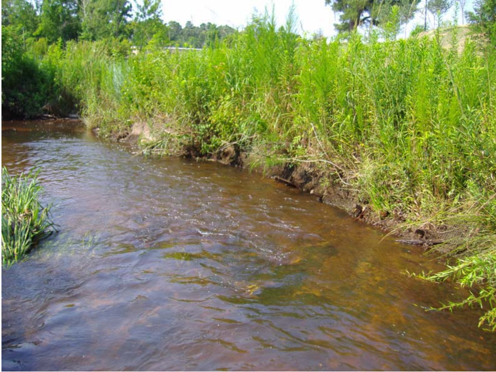
Photo 9. (SPA 5, 6, 8, 12, 14, 15, 17) Example of bank erosion (7/4/07)
