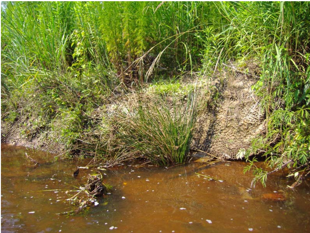
Photo 8. (SPA 1, 13, 18) Example of toe scouring around meandering bends (7/4/07)
