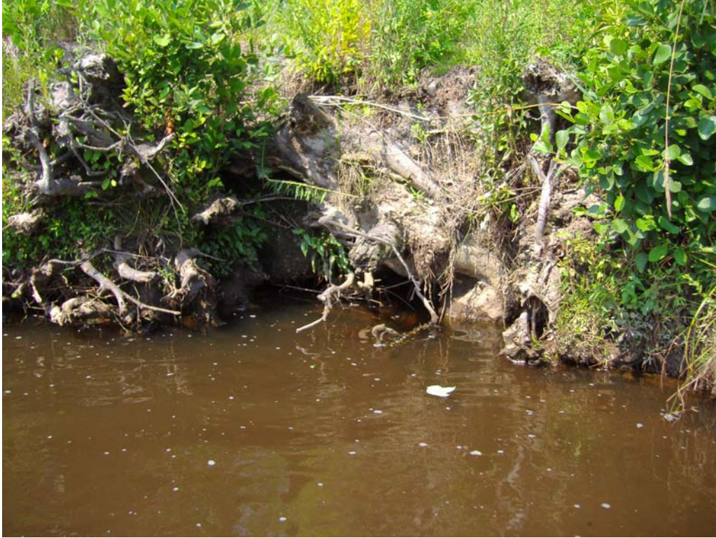
Photo 7. (SPA 7, 11, 19) Example of root wad failure - scouring around a root wad structure (7/4/07)
