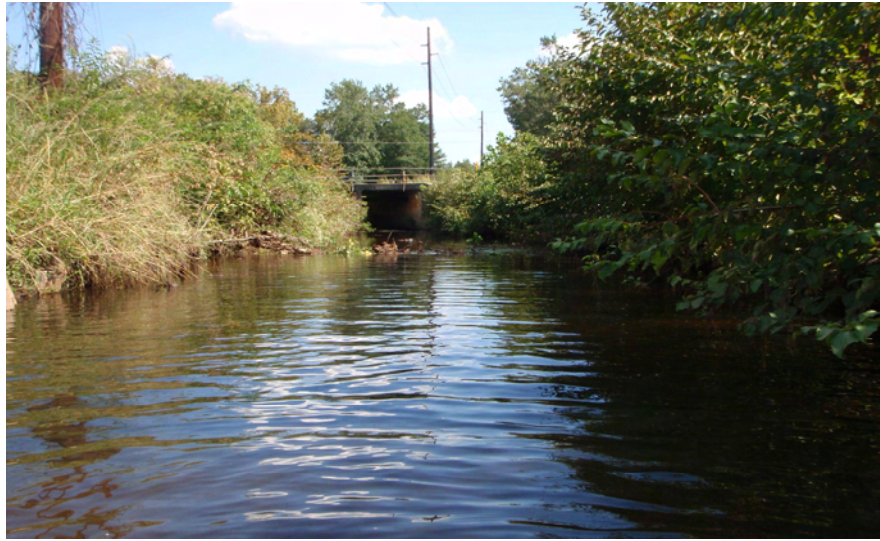
Photo of Cross-Section 4 - Reach 1 - Looking Downstream @ STA 23+05
