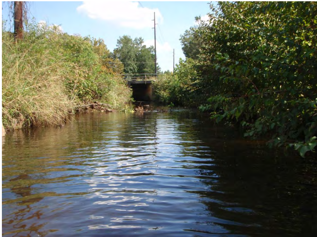
Photo Station 4 – Cross Section 4 looking downstream (9/16/10)
