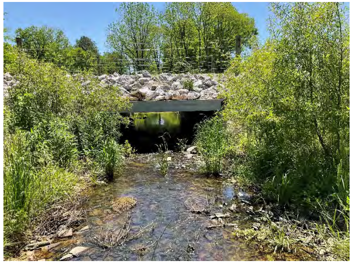
UT1 R2 – Looking Downstream (5/9/2023)
