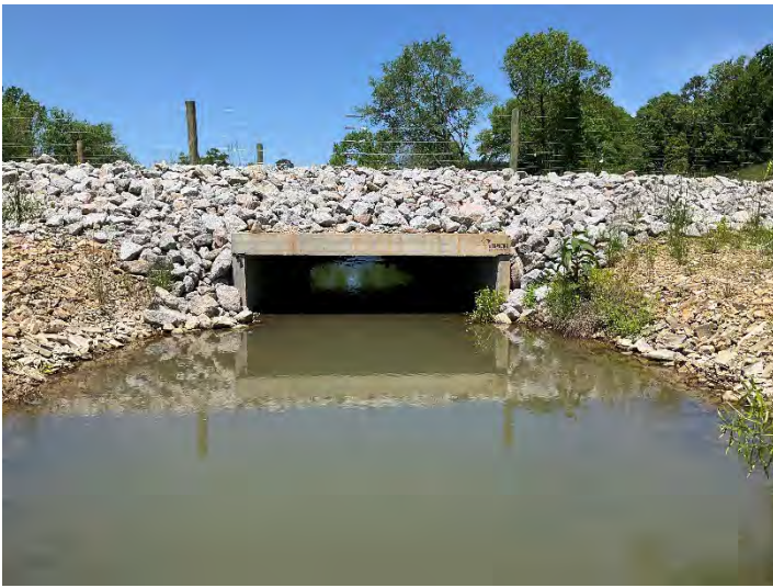
UT1 R2 – Looking Upstream (5/9/2023)
