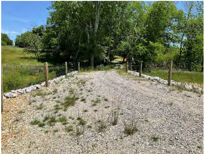
UT1 R2 Culvert Crossing – Looking Northeast (5/9/2023)
