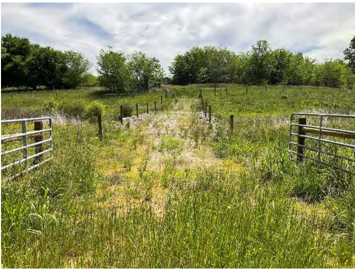
UT1B Culvert Crossing – Looking West (5/9/2023)
