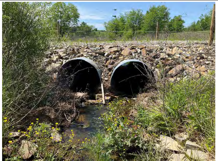
UT1B – Looking Downstream (5/9/2023)
