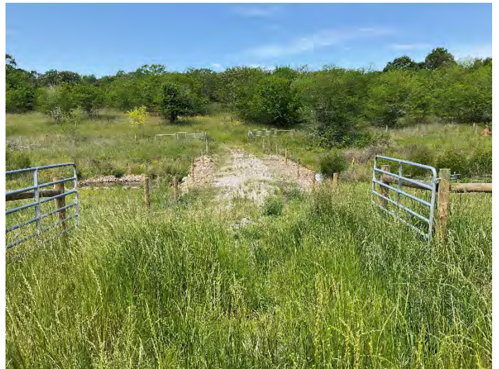
UT1B Culvert Crossing – Looking East (5/9/2023)
