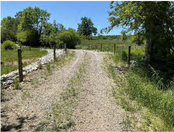
UT1 R2 Culvert Crossing – Looking Southwest (5/9/2023)
