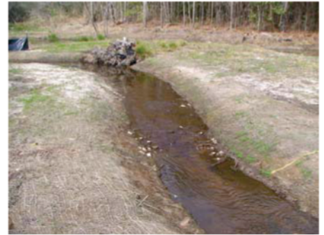
3/21/2007 Photo Point 3 Constructed Riffle 2
