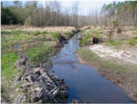
3/21/2007 Photo Point 1 Constructed Riffle 1
