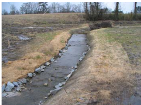
3/21/2007 Photo Point 22 Constructed Riffle 16
