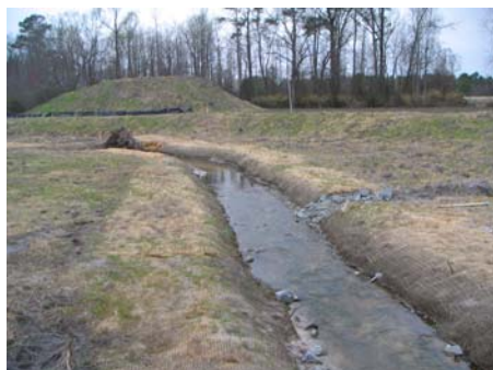
3/21/2007 Photo Point 23 Constructed Riffle 17
