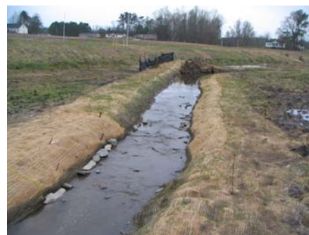
3/21/2007 Photo Point 18 Constructed Riffle 12
