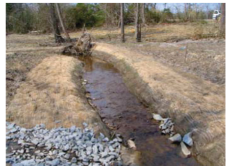
3/21/2007 Photo Point 9 Constructed Riffle 4
