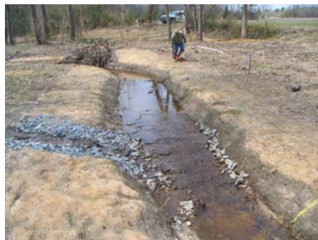
3/21/2007 Photo Point 11 Constructed Riffle 5
