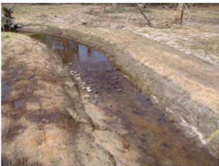
3/21/2007 Photo Point 7 Constructed Riffle 3
