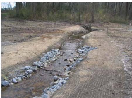
3/21/2007 Photo Point 13 Constructed Riffle 7
