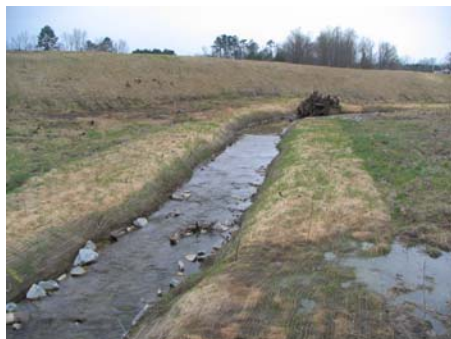
3/21/2007 Photo Point 20 Constructed Riffle 14
