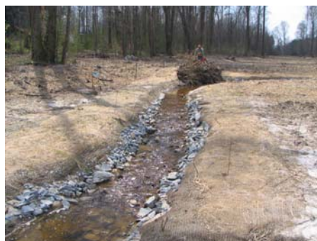
3/21/2007 Photo Point 17 Constructed Riffle 11
