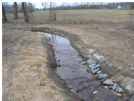
3/21/2007 Photo Point 14 Constructed Riffle 8
