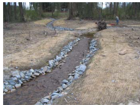
3/21/2007 Photo Point 15 Constructed Riffle 9
