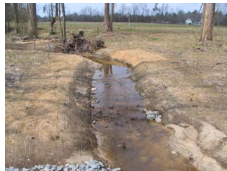
3/21/2007 Photo Point 12 Constructed Riffle 6
