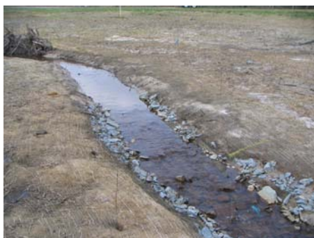
3/21/2007 Photo Point 16 Constructed Riffle 10
