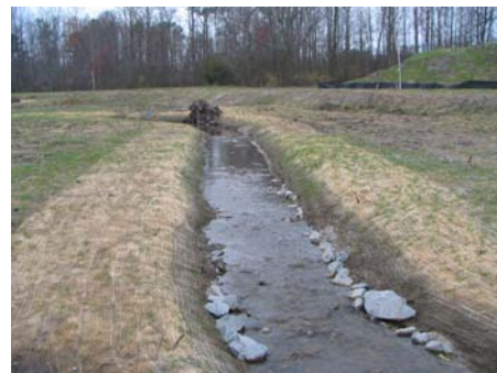
3/21/2007 Photo Point 21 Constructed Riffle 15
