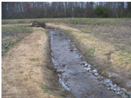
3/21/2007 Photo Point 19 Constructed Riffle 13
