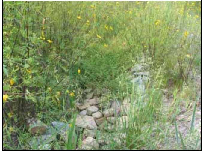
Photo Point 14 - Constructed Riffle 8
