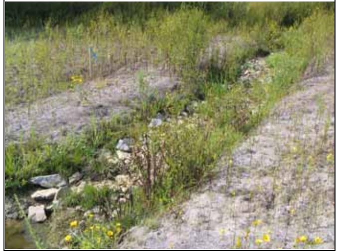
Photo Point 20 - Constructed Riffle 14
