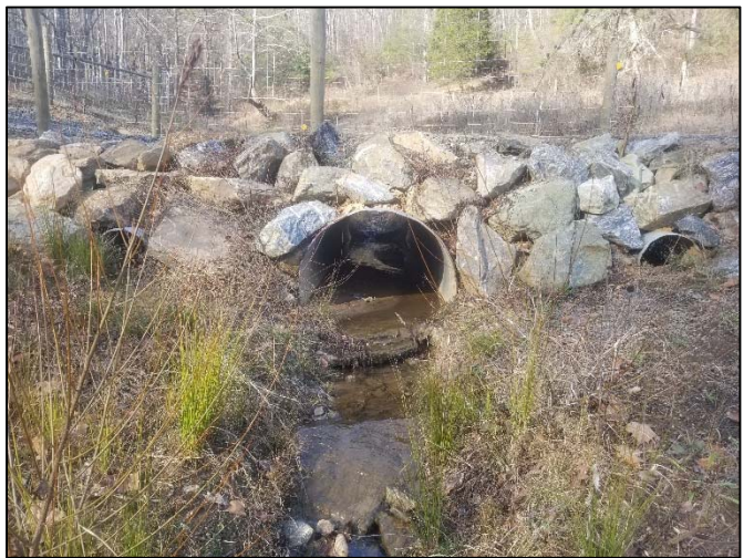
Culvert on T3 – 12/20/22
