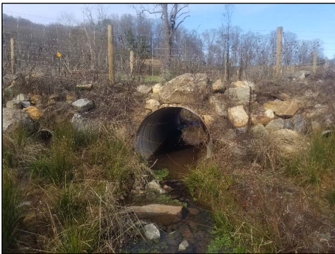
Culvert on T1 – 12/20/22
