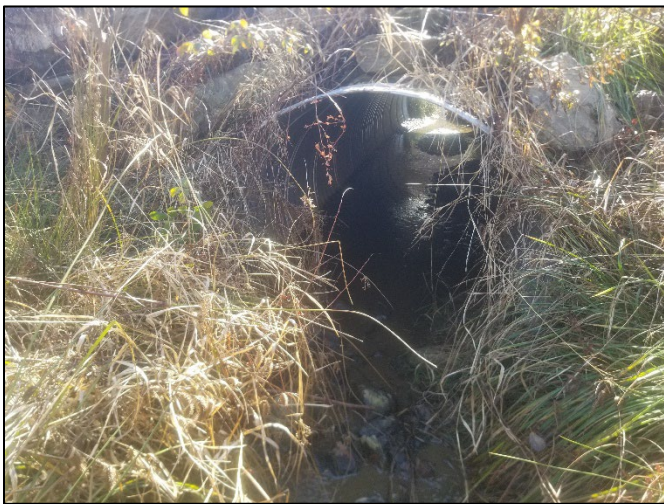
Culvert on T1 upstream – MY-02 – 12/11/23
