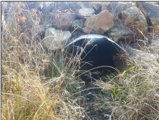
Culvert on T3 upstream – MY-02 – 12/11/23
