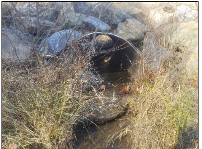
Culvert on T3 downstream – MY-02 – 12/11/23
