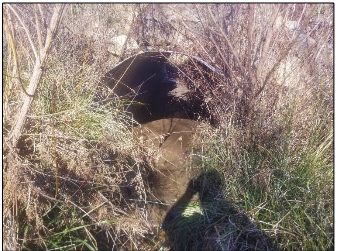
Culvert on T1 downstream – MY-02 – 12/11/23
