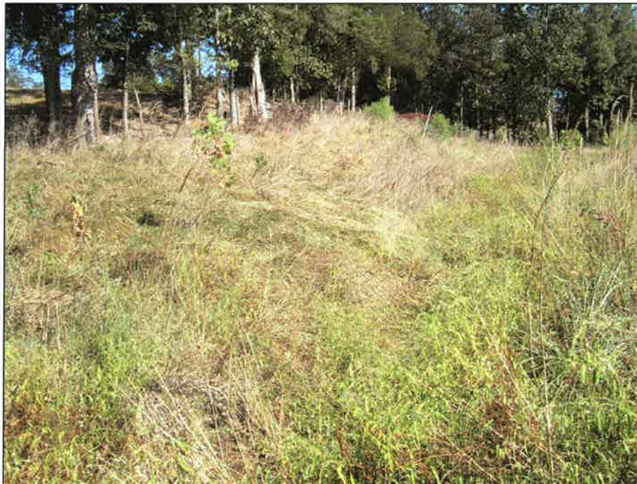
Fixed Station 6 Overview of Davis Branch, looking upstream near Station 38+75. (EMH&T, Inc. 9/20/10)
