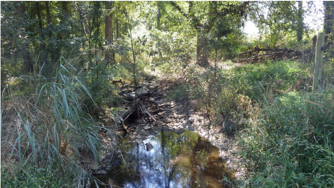
Fixed Station 4 Overview of Davis Branch, looking upstream near Station 25+75. (Top Photo – Year 1: Sept-2009, Bottom Photo – Year 5: 10/1/2013). (EMH&T)
