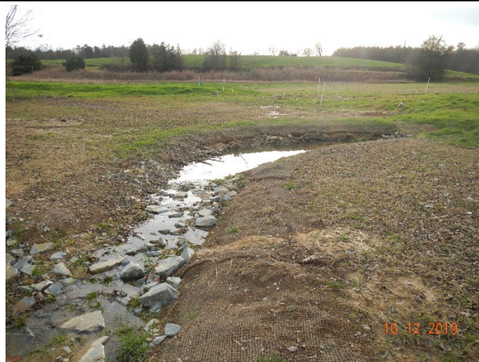
Photo Point 4 – WF2 Confluence, view upstream (12/16/2019)
