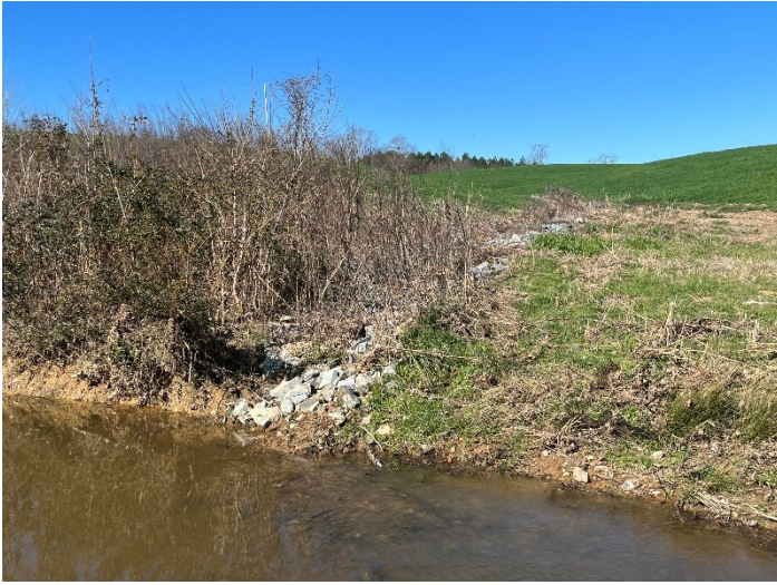
Meadow Branch, station 107+10 – Repaired gully (02/06/2023)
