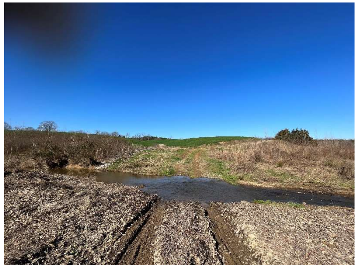
Ford Crossing Photo – Meadow Branch, looking west (02/06/2023)
