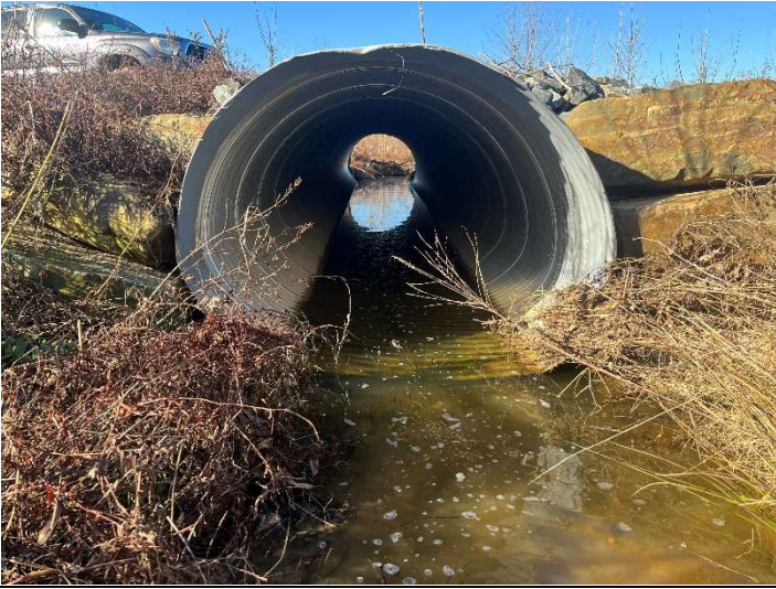
Culvert Photo – EF1, inlet (02/06/2023)
