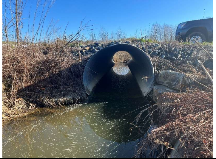
Culvert Photo – EF1 outlet (02/06/2023)
