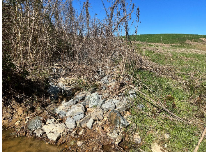
Meadow Branch, station 107+10 – Repaired gully (02/06/2023)
