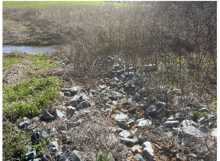
Meadow Branch, station 107+10 – Repaired gully (02/06/2023)
