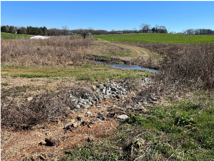
Meadow Branch, station 107+10 – Repaired gully (02/06/2023)
