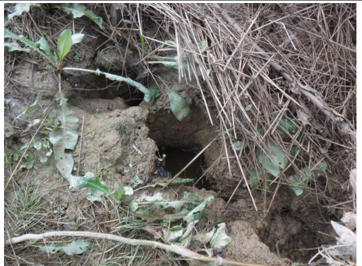
EF1 Issue: Bank Eroding behind structure 211+70- 212+00 (11/13/2020)
