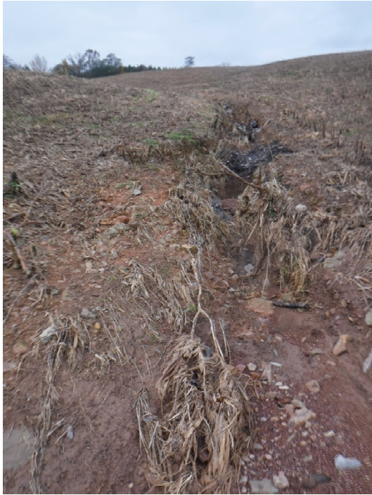
Scoured channel running from agricultural field into CE before flowing into Meadow Branch near station 107+50 (11/13/2020)
