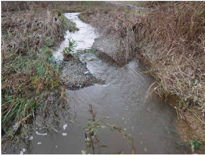
Issue: WF2 channel crossing being washed down stream causing aggradation (11/13/2020)
