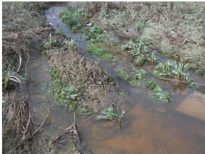
EF1 Vegetation in Channel at Station 212+70 (11/13/2020)
