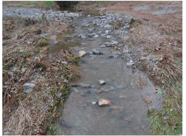
Issue: WF2 channel crossing being washed down stream causing aggradation (11/13/2020)
