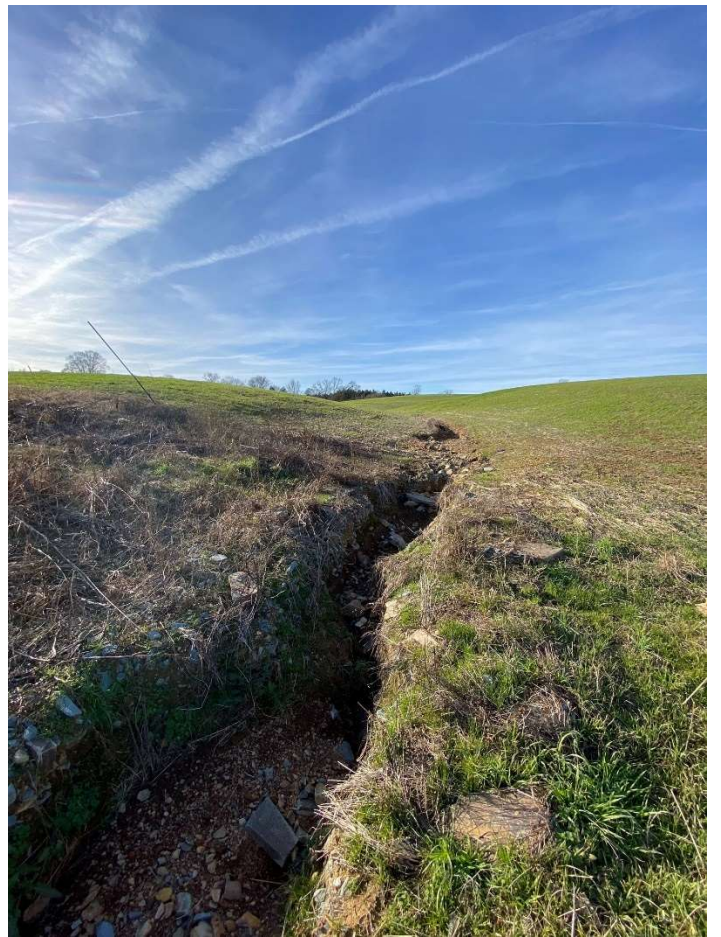
Meadow Branch: Partially filled in erosion gully outside of CE at 107+50 (01/12/2022)
