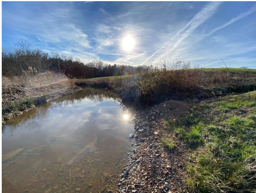
Meadow Branch: Deposition from partially filled in erosion gully into Meadow Branch at 107+50 (01/12/2022)
