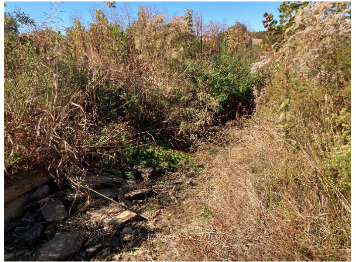
Photo Point 16 – EF1, view downstream (10/19/2021)
