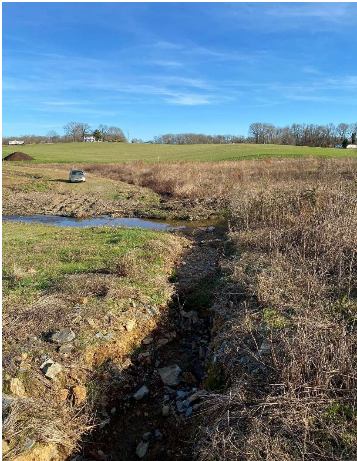
Meadow Branch: Partially filled in erosion gully outside of CE at 107+50 (01/12/2022)
