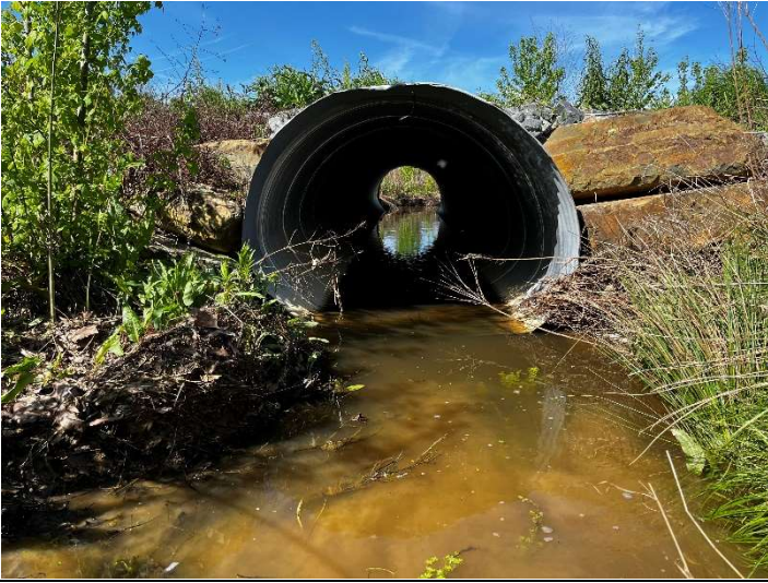
Culvert Photo – EF1, inlet (04/10/2023)
