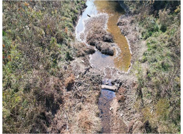
Meadow Branch, station 101+80, aerial photo – Recurring beaver dam and associated aggradation (11/7/2023)
