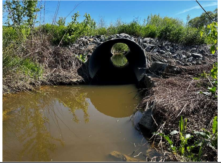
Culvert Photo – EF1 outlet (04/10/2023)
