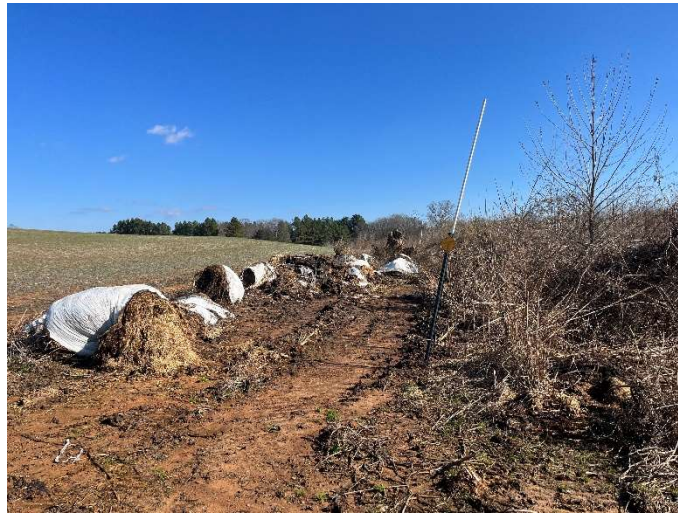
Between Easement Corners 2 and 3 – Hay bales removed from easement boundary (01/04/2024)
