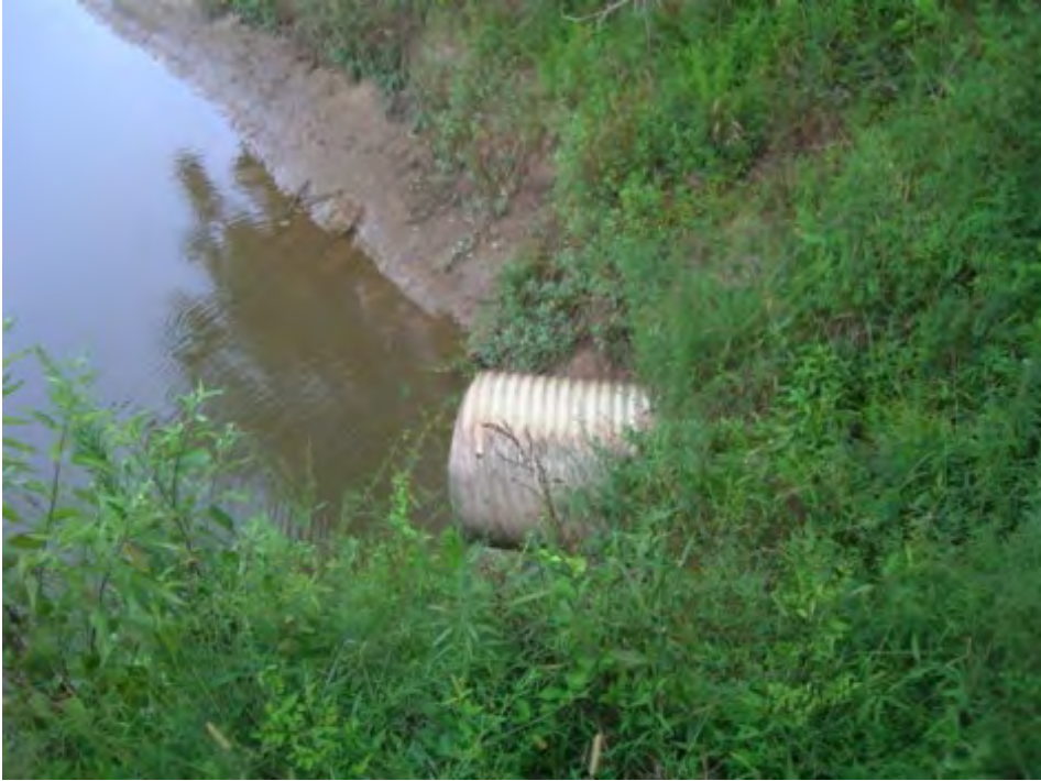
Outlet of Drop Structure at Downstream End of Project
