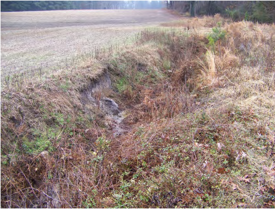
Existing conditions of upstream end of Southwest Branch
