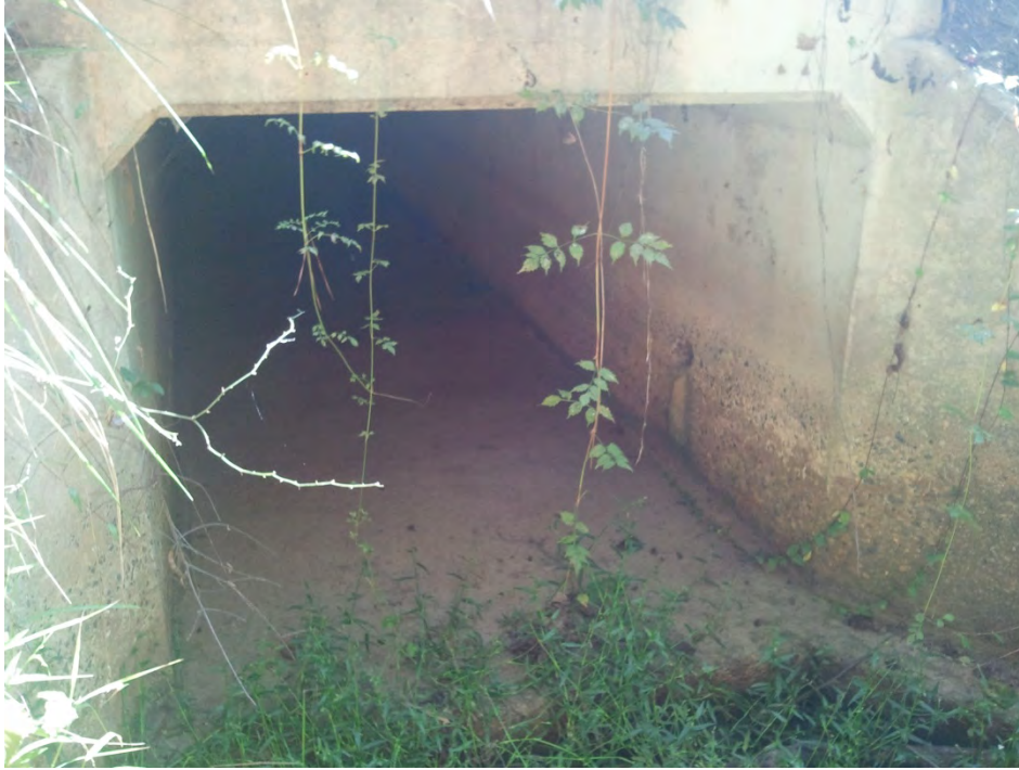
Culvert under U.S. Highway 701
