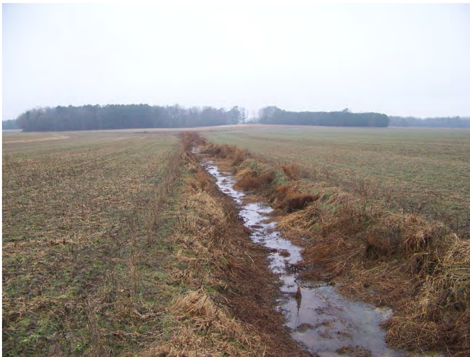
Existing conditions of Southeast Branch
