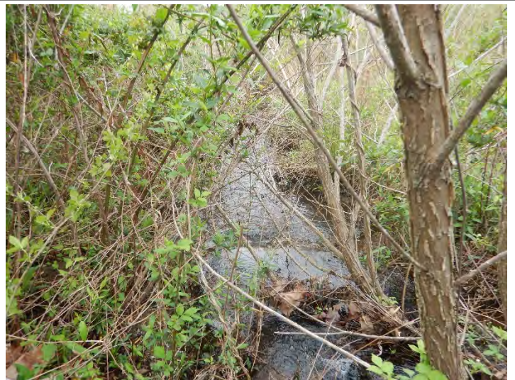
PHOTO POINT 14 DRT West - downstream (04/01/2020)
