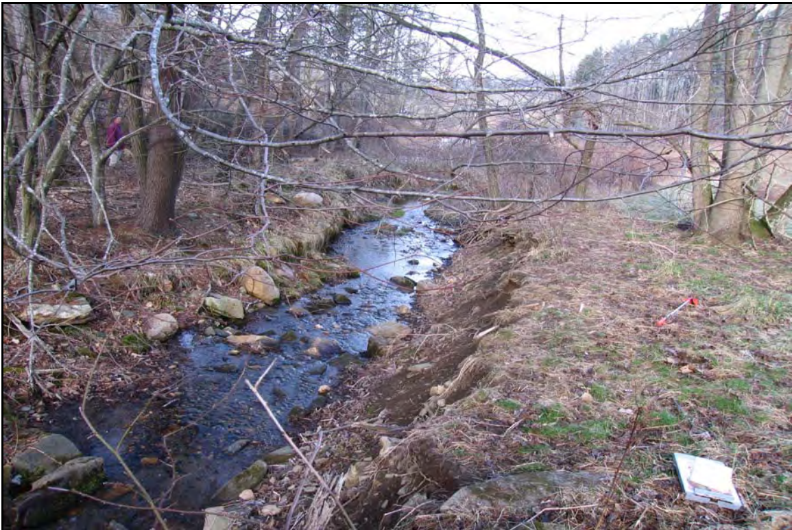
Poor riparian buffer and an eroding bank near the beginning of WOC-2.
