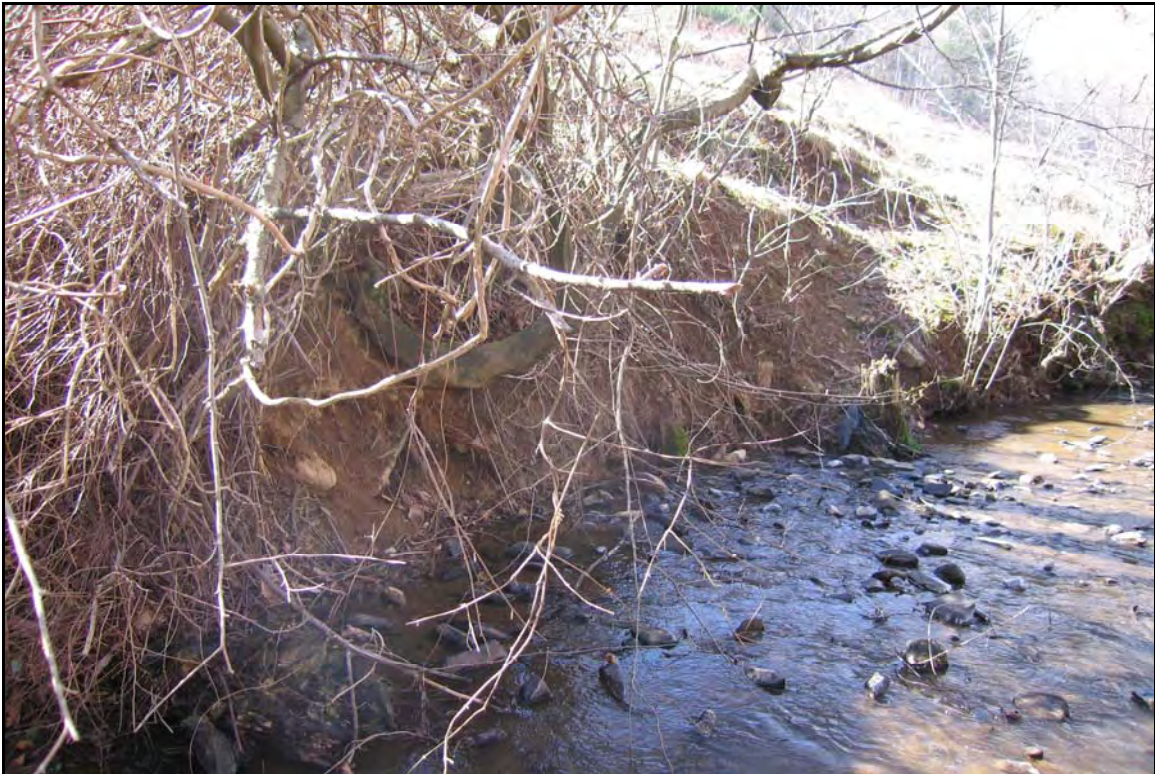
Bank erosion along WOC-4 after the confluence with T2.
