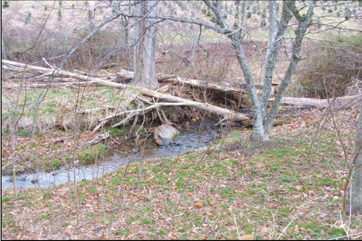
WOC-5 near the end of the project site.
