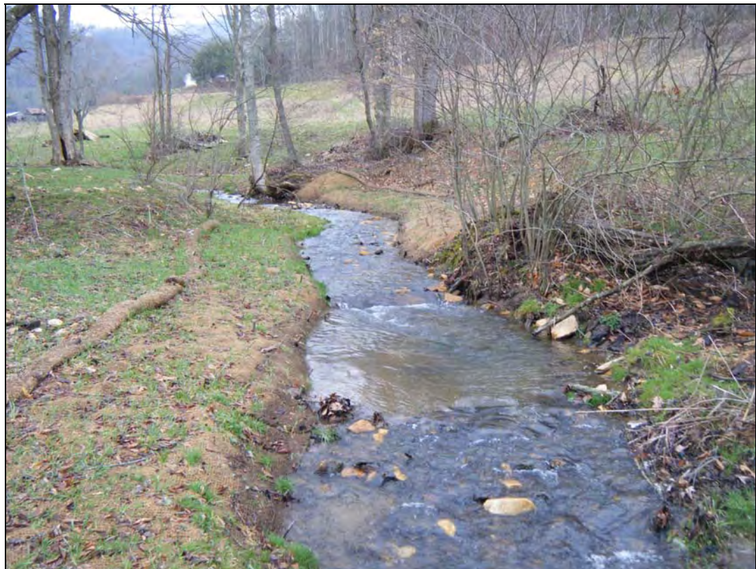
Photo Point 9: View looking upstream near Station 39+25. 3/23/10 – Baseline
