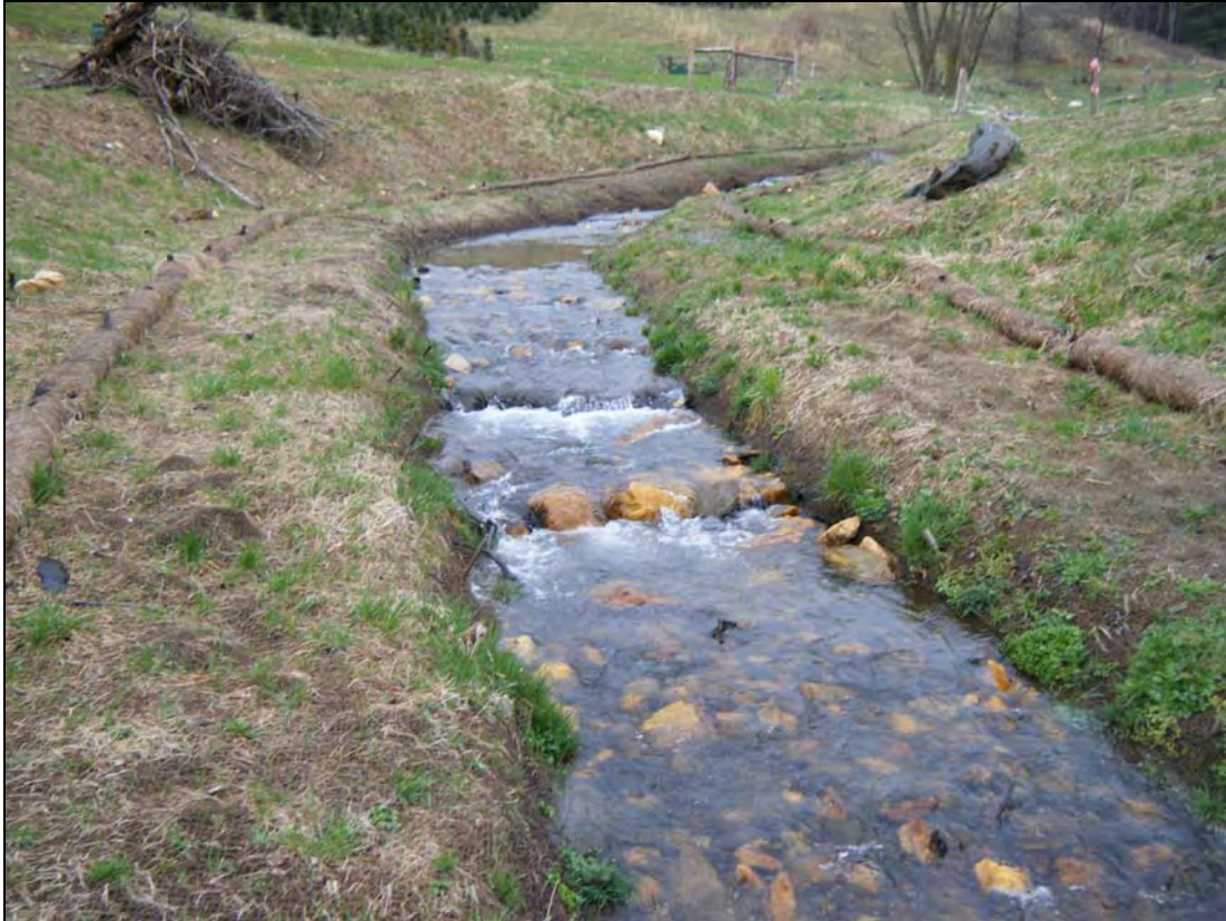
Photo Point 7: View looking upstream near Station 29+25. 3/23/10 – Baseline
