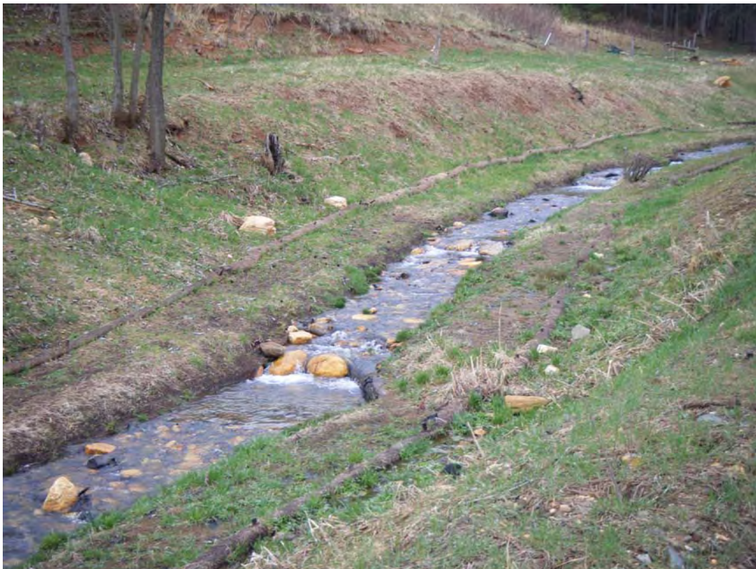
Photo Point 5: View looking upstream at WOC, near Station 26+25. 3/23/10 – Baseline
