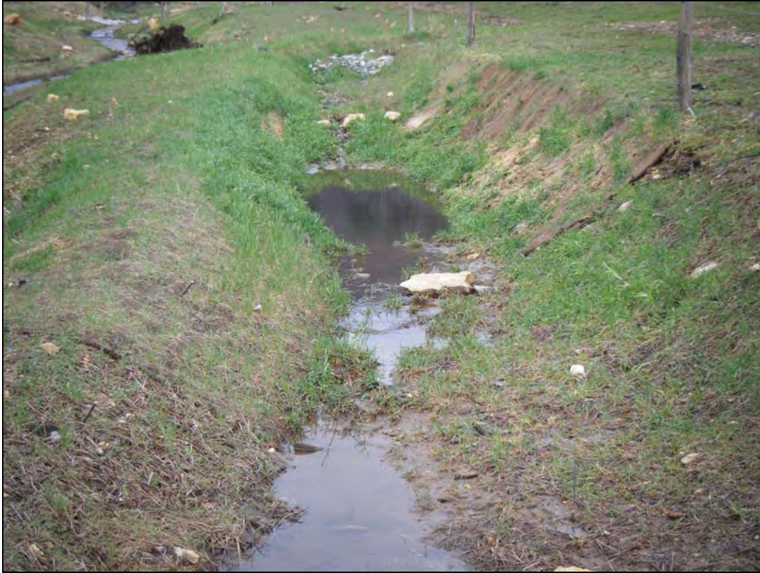
Photo Point 5: View looking at water treatment pool, near Station 26+25. 3/23/10 – Baseline
