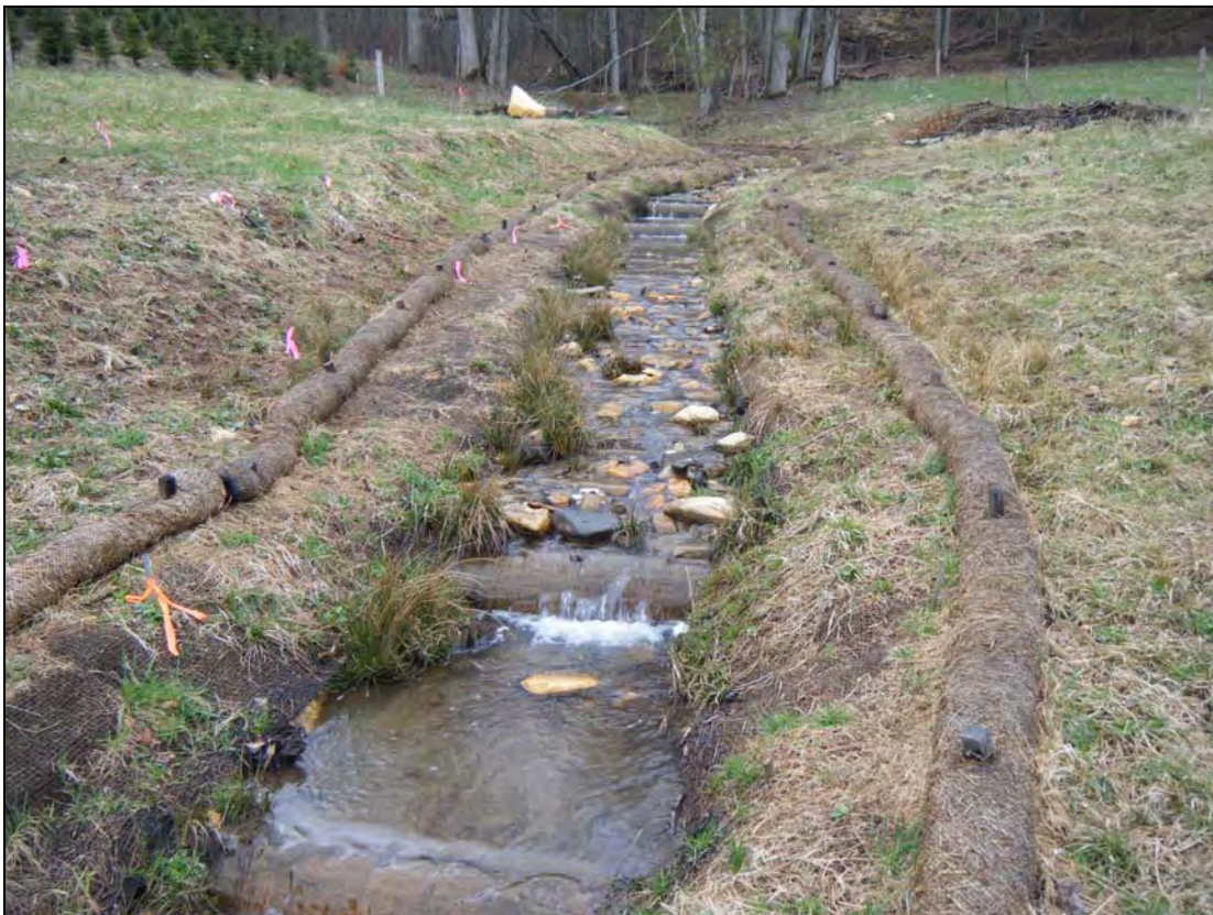
Photo Point 11: View looking upstream on T1 near Station 52+50. 3/23/10 – Baseline
