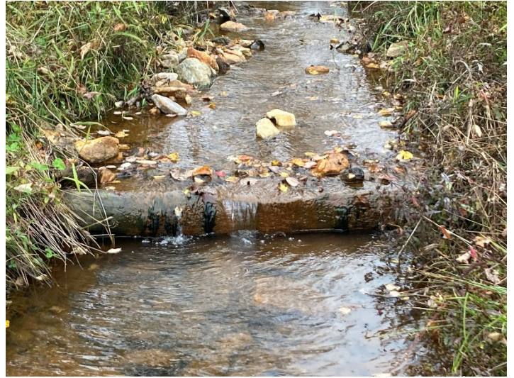
UT to Crab Creek R1 (113+46) – Piping Log Sill Repair (10/12/2022)
