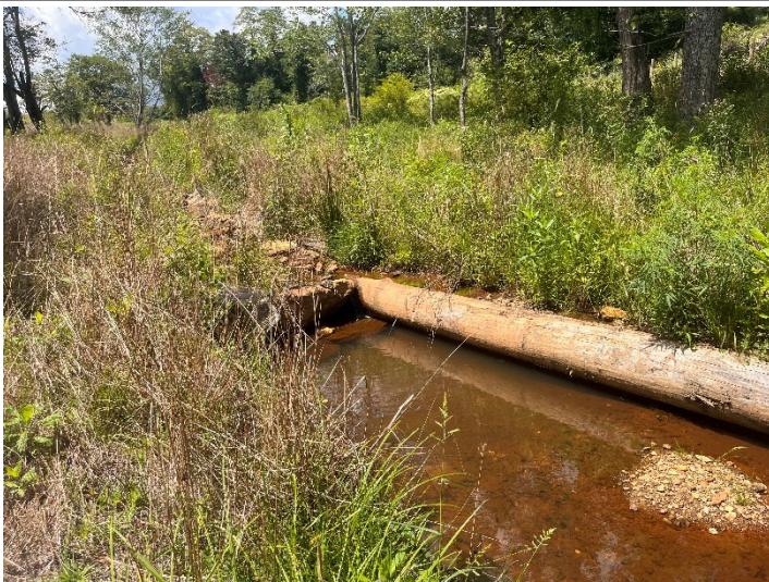
PHOTO POINT 6 UT to CC Reach 1 – upstream (8/9/2022)
