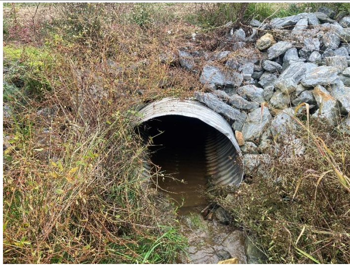
UT4 Reach 2 Crossing (413+54) – inlet (10/12/2022)
