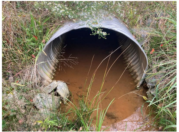
UT4 Reach 1 Crossing (404+74) – outlet (10/12/2022)
