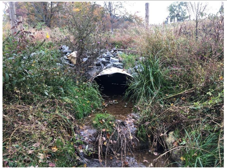
UT4 Reach 2 Crossing (413+96) – outlet (10/12/2022)
