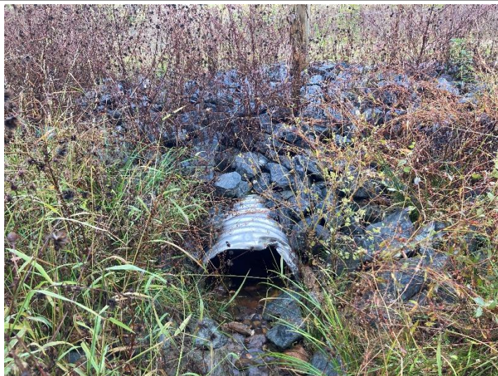
UT6 Crossing (605+26) – inlet (10/12/2022)
