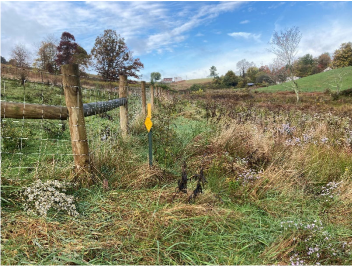
UT to Crab Creek R1 (Station 104+75 – 106+25) – Fence Relocated Outside of Conservation Easement (10/12/2022)
