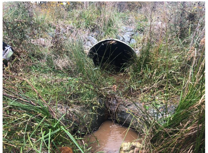
UT1A Reach 1 Crossing (155+17) – outlet (10/12/2022)
