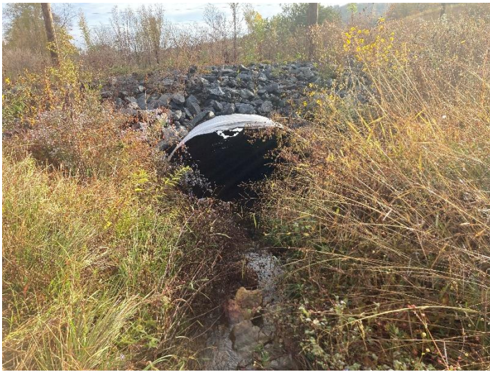
UT to Crab Creek Reach 1 Crossing 1 (102+83) – inlet (10/12/2022)
