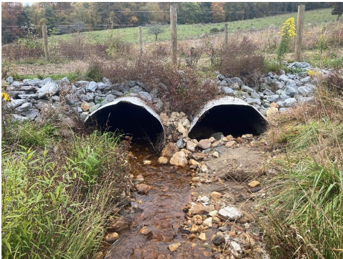
UT to Crab Creek R1 Crossing 2 (114+46) – inlet (10/12/2022)
