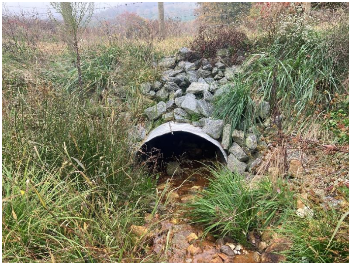
UT4 Reach 1 Crossing (404+33) – inlet (10/12/2022)
