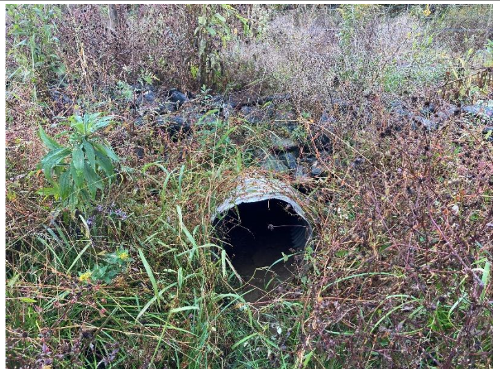
UT6 Crossing (605+71) – outlet (10/12/2022)
