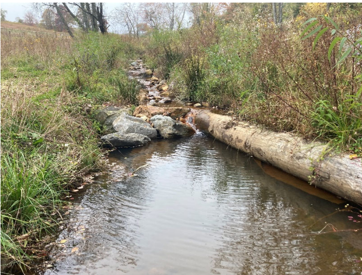
UT to Crab Creek R1 J-Hook (112+09) – Splash Rock Installation for AOP (10/12/2022)
