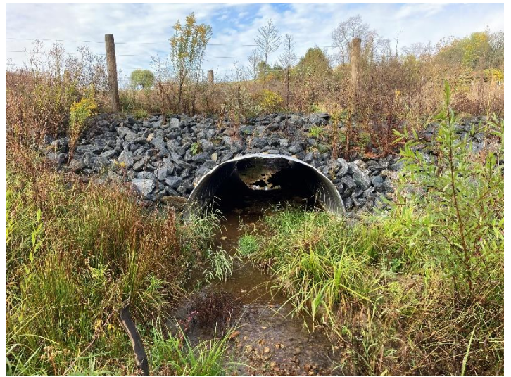
UT to Crab Creek Reach 1 Crossing 1 (103+33) – outlet (10/12/2022)
