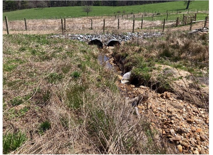
PHOTO POINT 7 UT to CC Reach 1 – downstream (4/3/2023)
