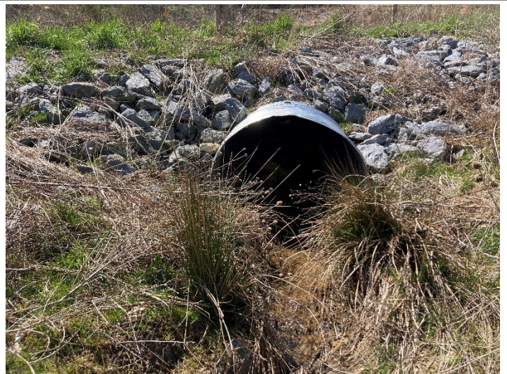
UT1A Reach 1 Crossing (155+17) – outlet (4/3/2023)
