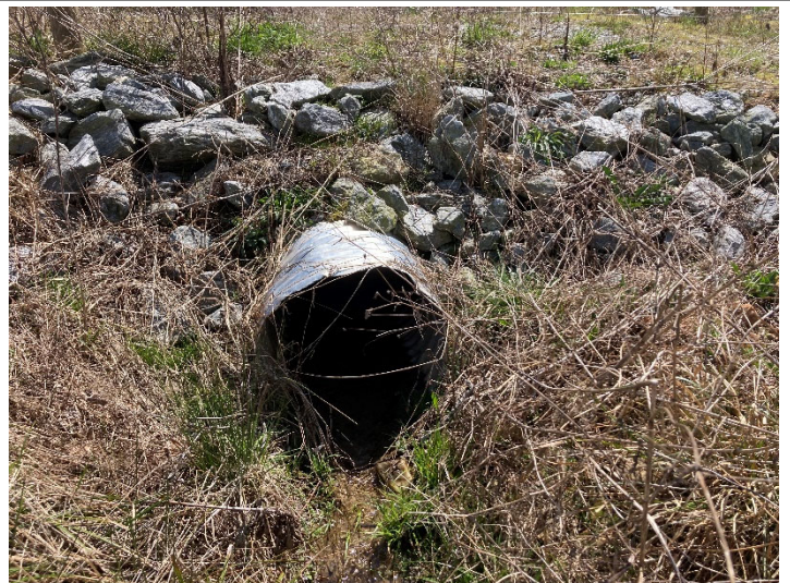
UT6 Crossing (605+71) – outlet (4/3/2023)
