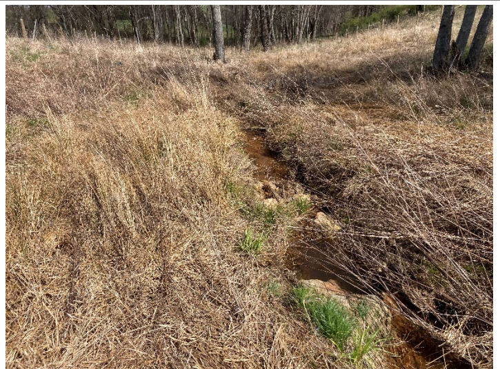
PHOTO POINT 27 UT1A Reach 1– downstream (4/3/2023)
