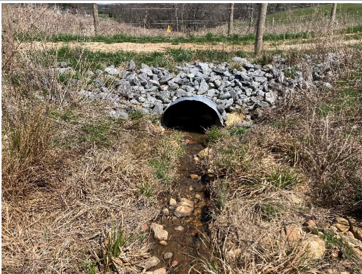
UT1A Reach 1 Crossing (154+73) – inlet (4/3/2023)
