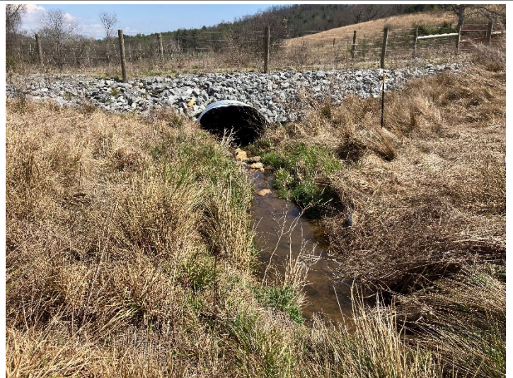
PHOTO POINT 3 UT to CC Reach 1 – downstream (4/3/2023)
