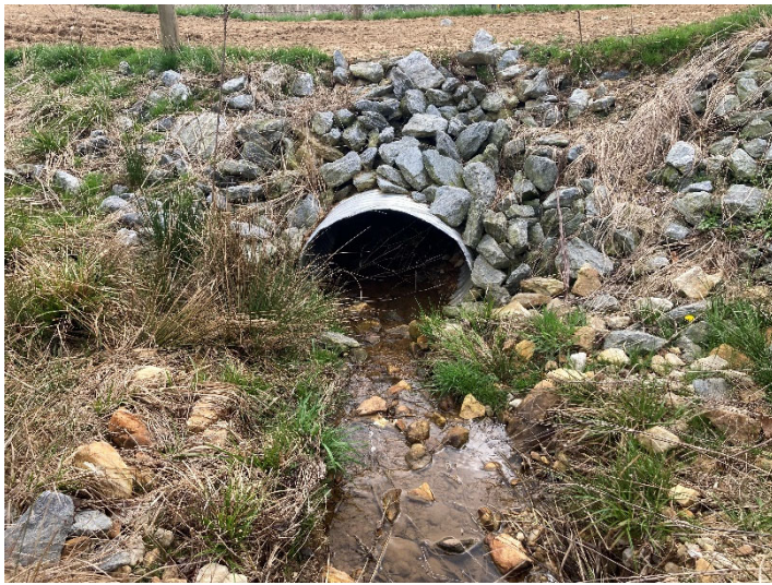
UT4 Reach 1 Crossing (404+33) – inlet (4/3/2023)
