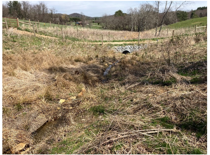
PHOTO POINT 26 UT1A Reach 1– downstream (4/3/2023)
