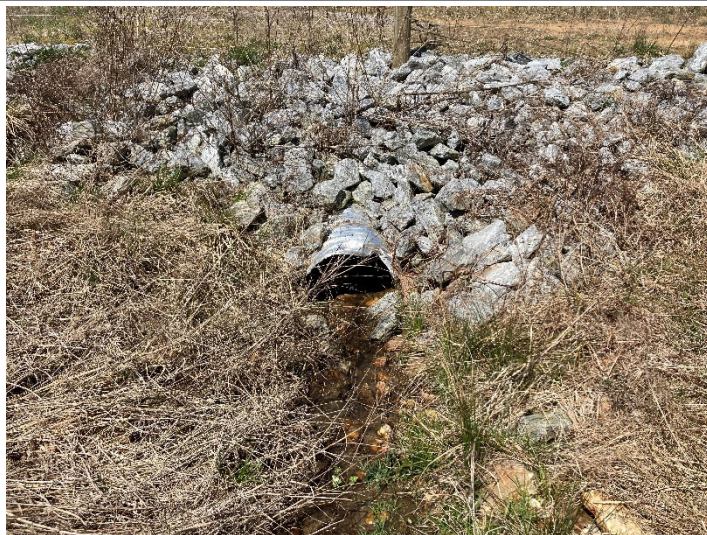
UT6 Crossing (605+26) – inlet (4/3/2023)
