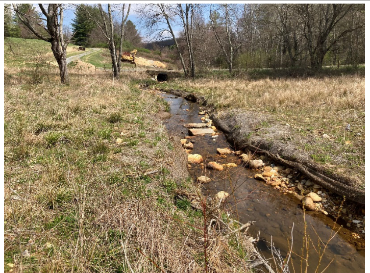
PHOTO POINT 12 UT to CC Reach 2 – downstream (4/3/2023)
