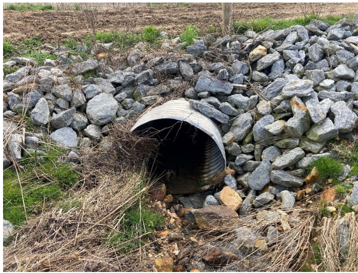
UT4 Reach 2 Crossing (413+54) – inlet (4/3/2023)
