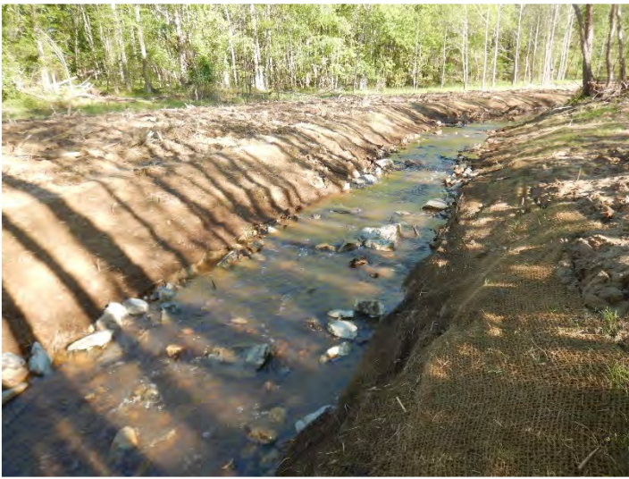
PHOTO POINT 16 Dry Creek R4 – upstream (04/27/2020)
