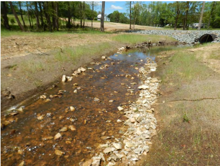
PHOTO POINT 5 Dry Creek R2 – upstream (04/27/2020)
