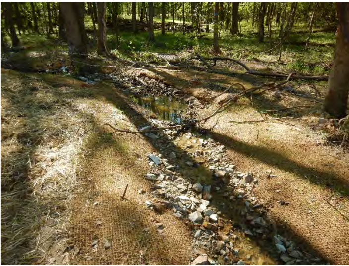
PHOTO POINT 29 UT6 R1 – upstream (04/27/2020)
