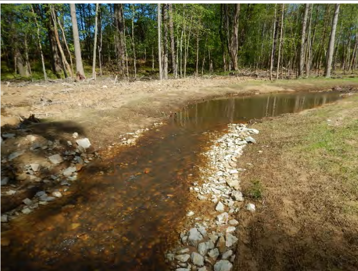
PHOTO POINT 12 Dry Creek R3 – upstream (04/27/2020)
