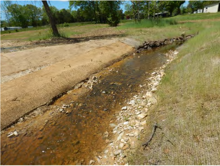
PHOTO POINT 1 Dry Creek R1 – upstream (04/27/2020)
