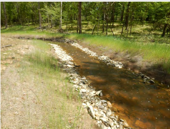
PHOTO POINT 6 Dry Creek R2 – upstream (04/27/2020)
