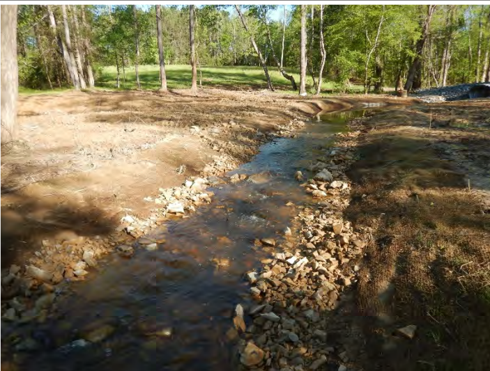
PHOTO POINT 15 Dry Creek R4 – upstream (04/27/2020)
