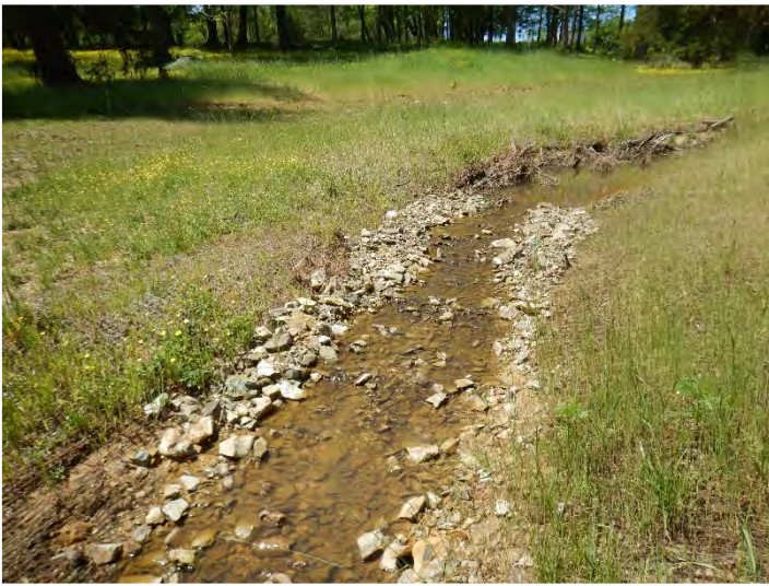
PHOTO POINT 19 UT1 R2 – upstream (04/27/2020)
