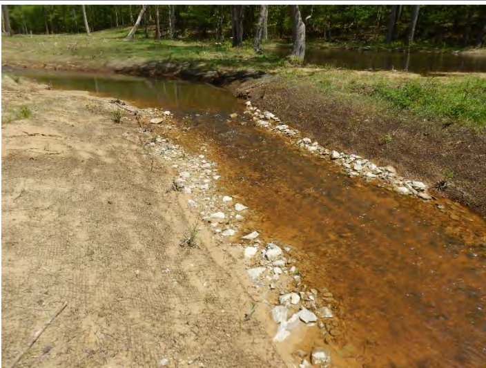
PHOTO POINT 9 Dry Creek R2 – upstream (04/27/2020)
