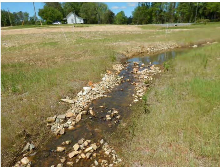
PHOTO POINT 21 UT1 R2 – upstream (04/27/2020)
