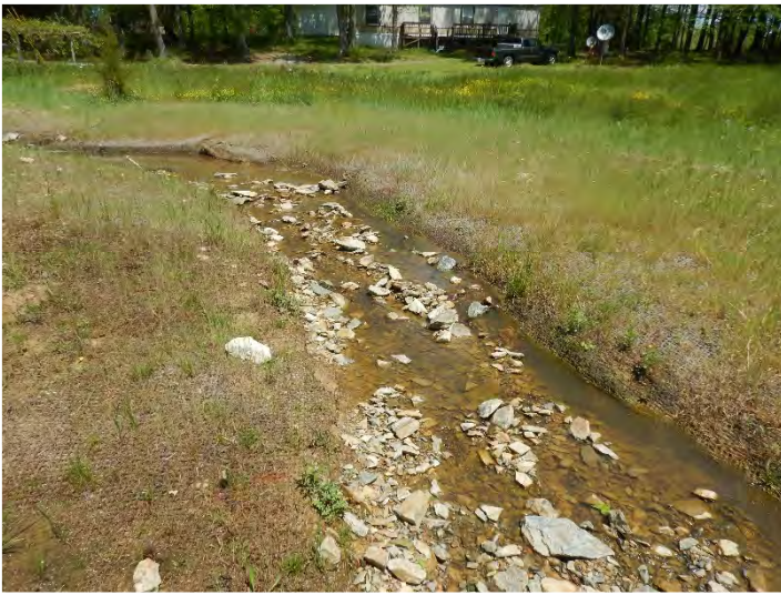
PHOTO POINT 20 UT1 R2 – upstream (04/27/2020)
