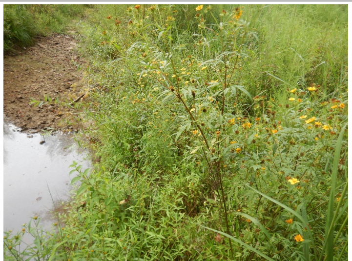
After – Repaired Localized Erosion (09/16/2021)
