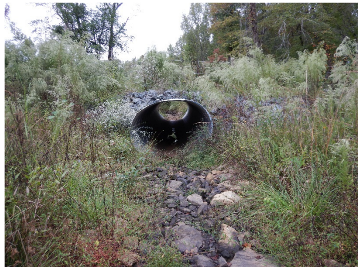
Dry Creek Reach 4 – Looking Downstream (10/12/2021)
