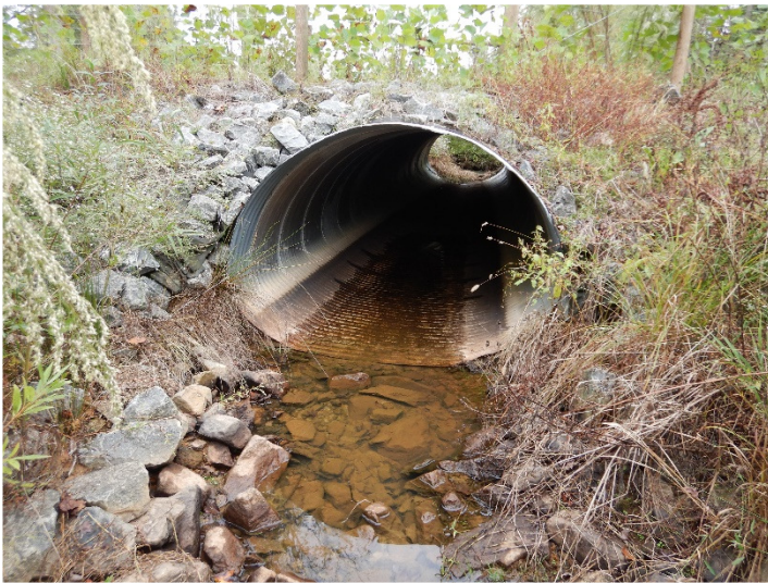
Dry Creek Reach 2 – Looking Upstream (10/12/2021)
