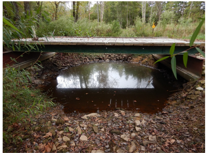
Dry Creek Reach 2 – Looking Downstream (10/12/2021)
