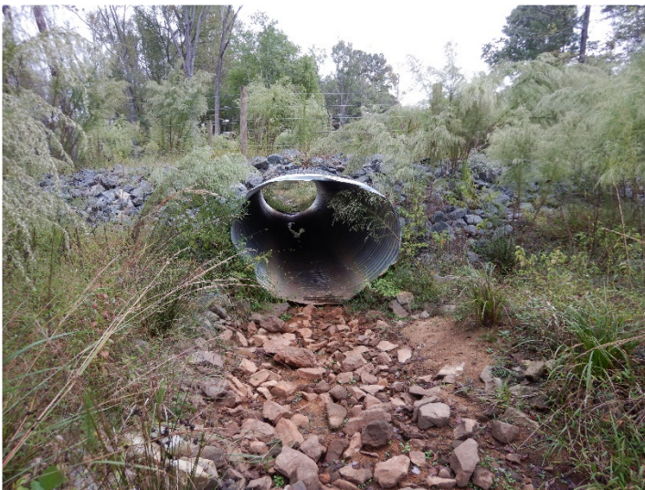
Dry Creek Reach 4 – Looking Upstream (10/12/2021)
