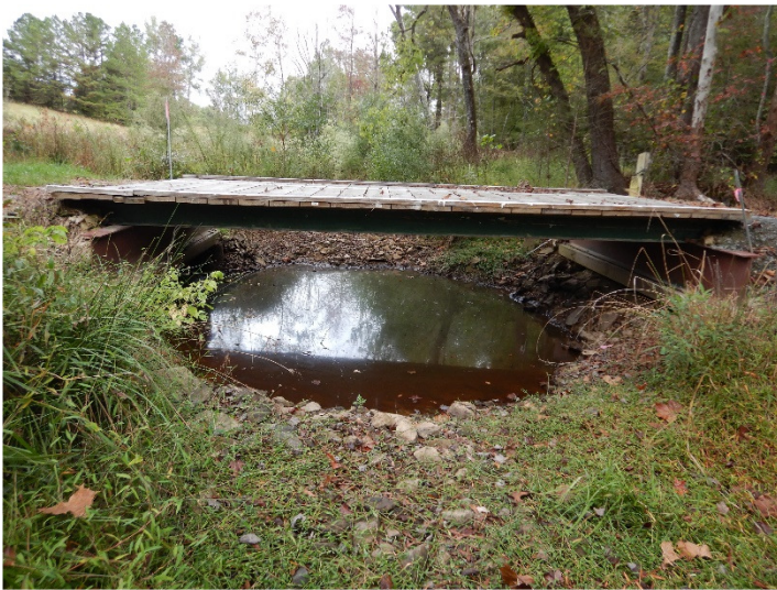
Dry Creek Reach 2 – Looking Upstream (10/12/2021)
