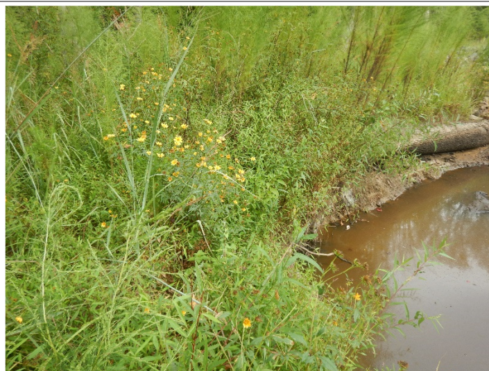
After – Repaired Localized Erosion (09/16/2021)
