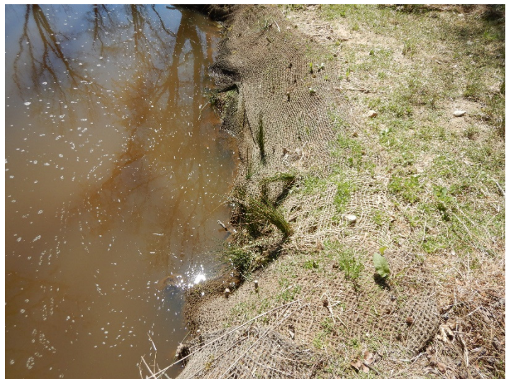
After – Repaired Localized Erosion (04/2/2021)
