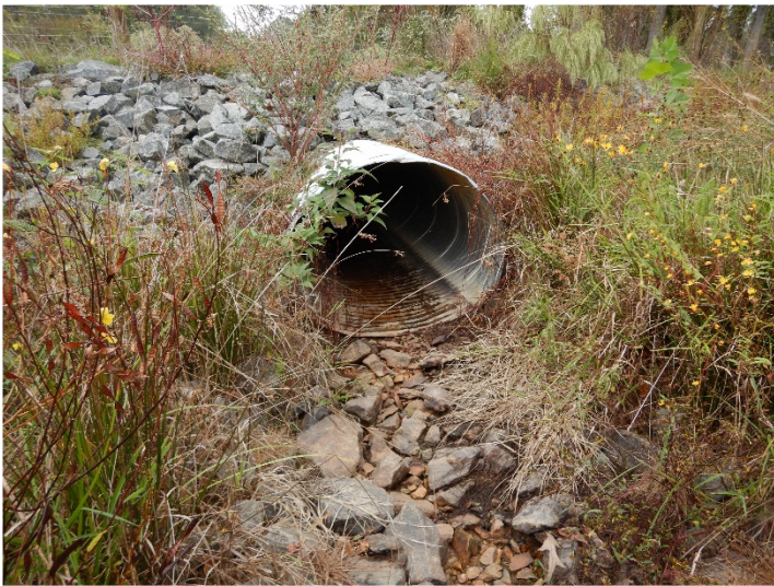
UT1 Reach 2 – Looking Upstream (10/12/2021)
