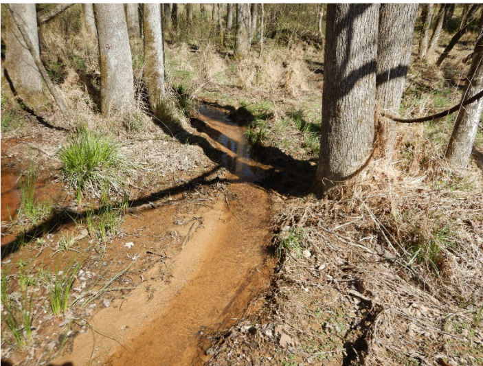
PHOTO POINT 31 UT6 R2 – upstream (4/2/2021)
