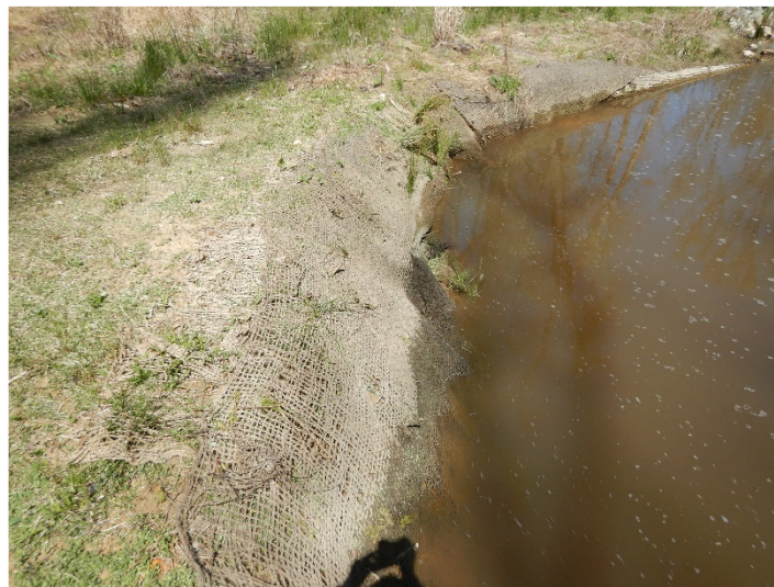
After – Repaired Localized Erosion (04/2/2021)
