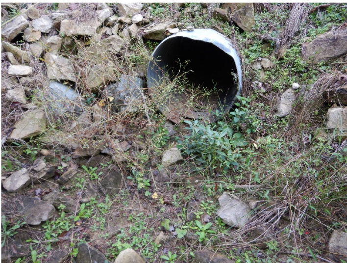
UT5 – Looking Upstream (10/12/2021)
