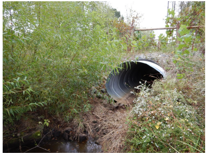
Dry Creek Reach 2 – Looking Downstream (10/12/2021)
